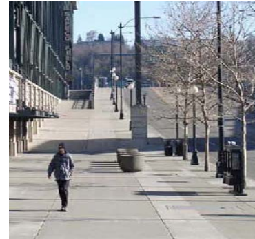
New South Atlantic Street overpass built in SR 519 Phase 1
