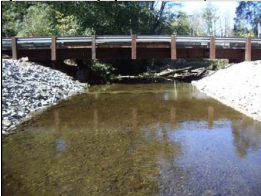
Figure 9-4 Culvert to bridge replacement, Shine Estuary.
