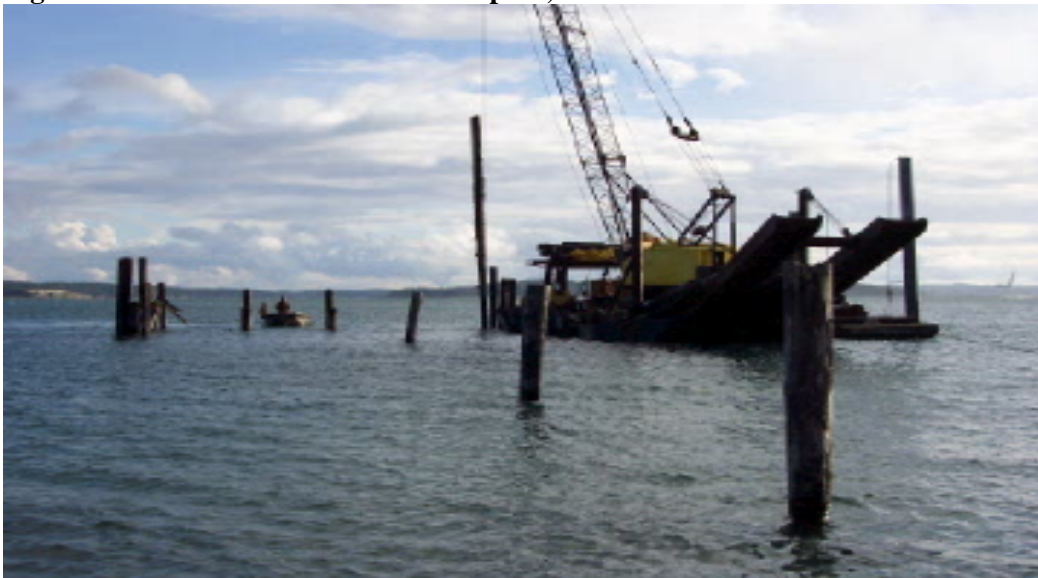
Figure 12-3 Removal of creosote wood piles, Northwest Maritime Center Dock.
