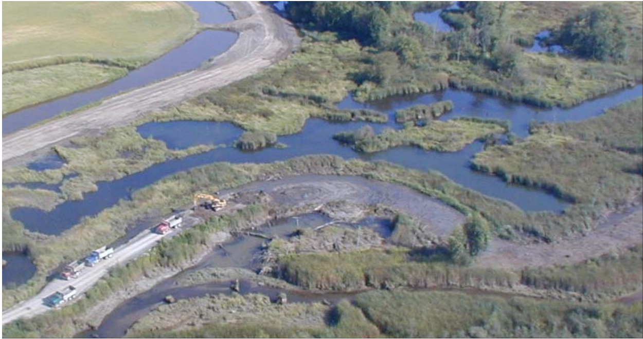
Figure 3-3. Reconnection of remnant channel with outboard channel by excavation through the dike foundation (Hood 2004)
