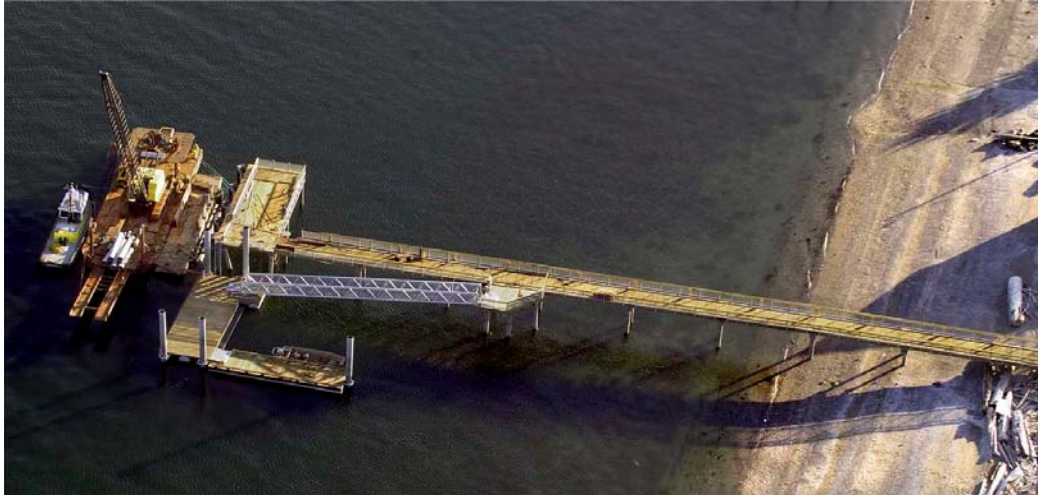
Figure 12-2 Extended and reoriented pier, Northwest Maritime Center Dock.
