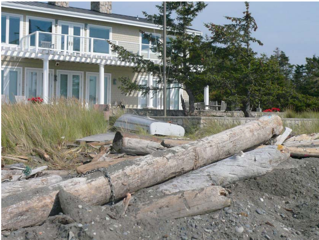
Figure 11-3 Anchored LWD project for erosion control immediately after installation in 2008 (Coastal Geologic Services).
