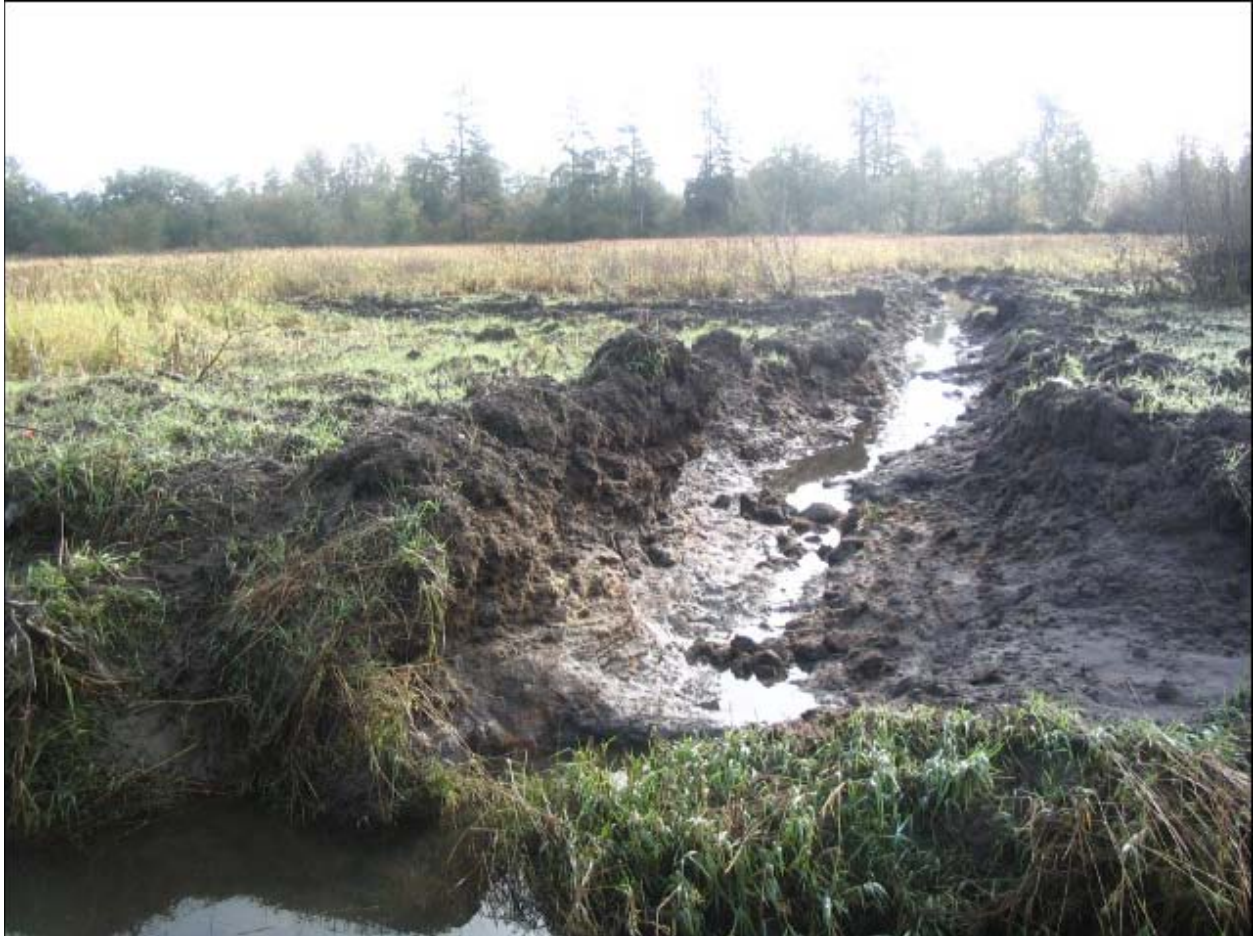
Figure 4-3. Milltown Island tidal channel created with explosives.
