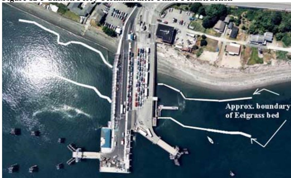
Figure 12-5 Clinton Ferry Terminal after Phase I construction
