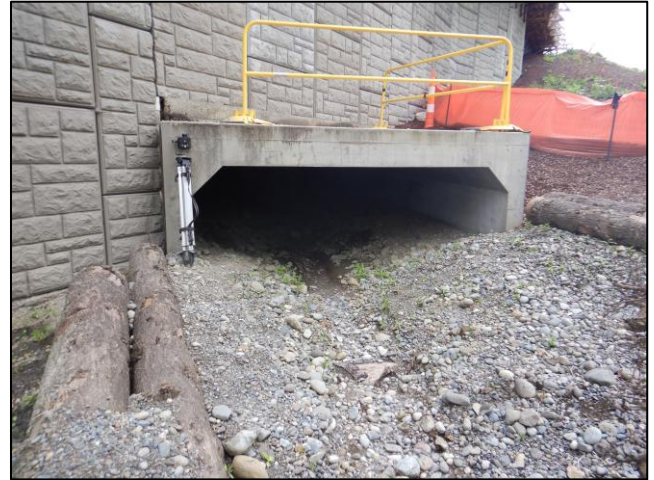
Figure 13. 932933 After Construction: The project replaced the two culverts with a single 427 ft long box culvert. The box culvert has a span of 12 ft and a rise of 8.0 ft.
