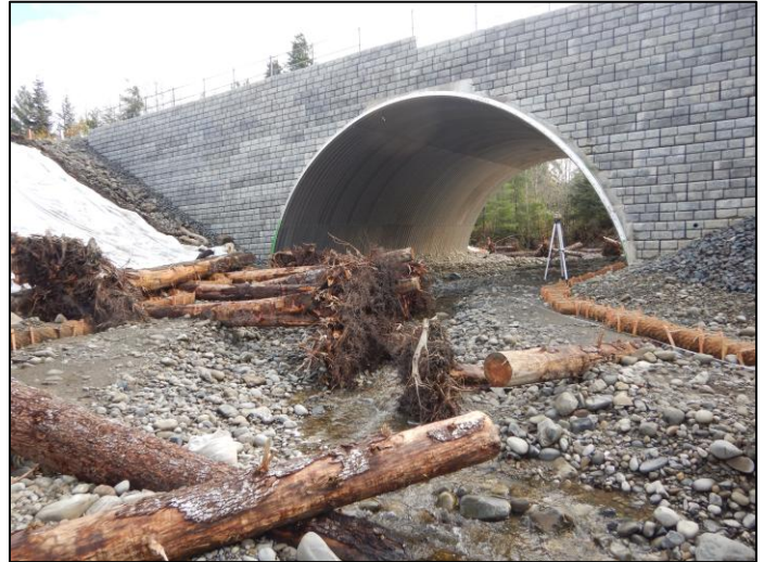
Figure 64. 991507 After Construction: The new crossing is a 41 ft span by 27 ft rise aluminum, bottomless arch culvert.
