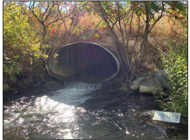
Figure 90. 990217 Before Construction: The old crossing was a squashed corrugated steel culvert with a 6 ft span, 4ft rise and 100 ft long. The old crossing was a barrier due to hydraulic drop.
