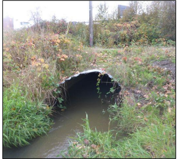
Figure 21. 935093 Before Construction: The crossing consisted of a 184.5 ft long squashed culvert with a span of 8.5 ft and a rise of 6 ft. During the previous site assessment, it was determined that this site was not a barrier to fish passage. The crossing was filled and abandoned in place beneath new highway infrastructure.
