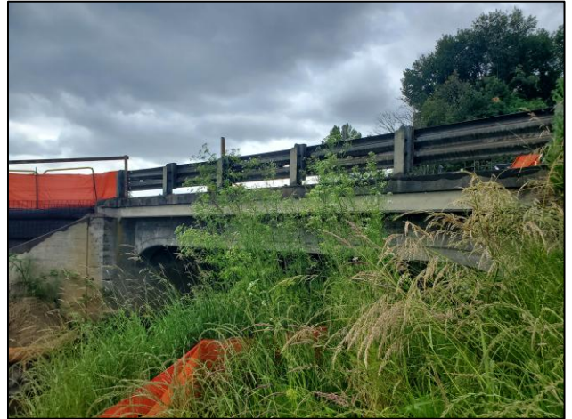
Figure 31. 921131 Before Construction: The previous fish passable bridge was built in 1927 and rebuilt in 1953.
