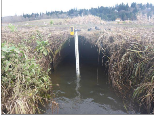
Figure 22. 935157 Before Construction: This crossing was a single corrugated steel squashed culvert with a span of 4 ft and a rise of 4.5 ft. The culvert length was 20 ft long and provided access to a large agricultural area. The culvert was a barrier to fish passage due to excessive slopes.
