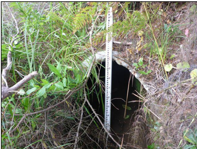
Figure 69. 997780 Before Construction: The old crossing was a 3 ft diameter concrete culvert and was a barrier due to slope.
