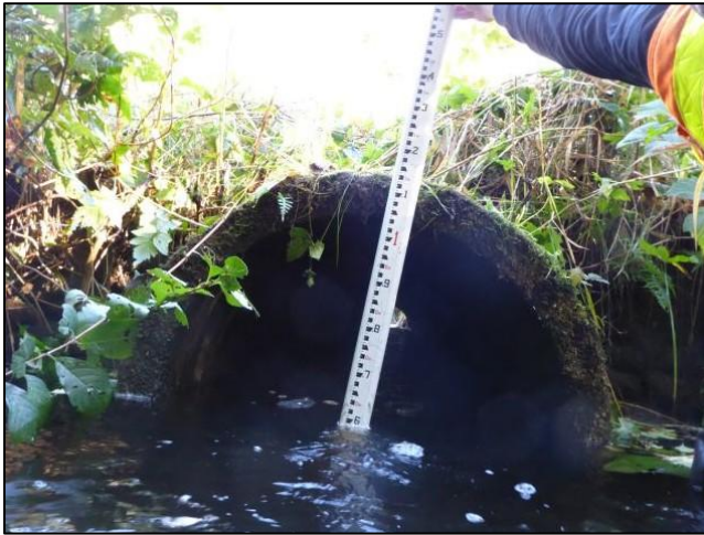
Figure 65. 990920 Before Construction: The old crossing was a 3 ft diameter concrete culvert that was assessed as a slope barrier.
