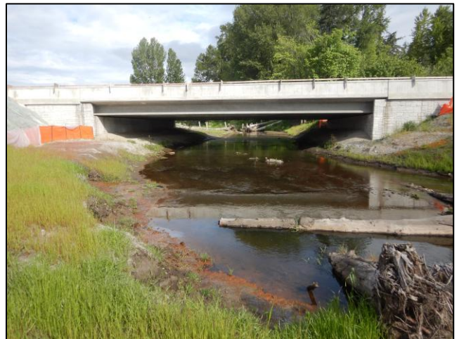
Figure 32. 921131 After Construction: The new, concrete bridge is 69 ft long and includes a wildlife bench on one side.
