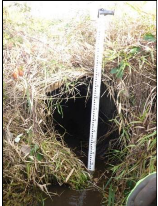
Figure 29. 921588 Before Construction: This crossing was a corrugated steel culvert with a diameter of 3 ft. This culvert was 36 ft long and provided conveyance under an agricultural field access road.
