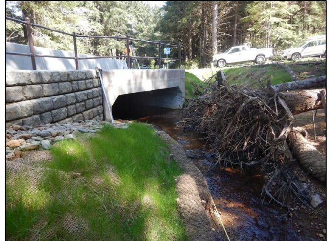
Figure 70. 997780 After Construction: The new crossing is a 14 ft span by 9 ft rise concrete box culvert.
