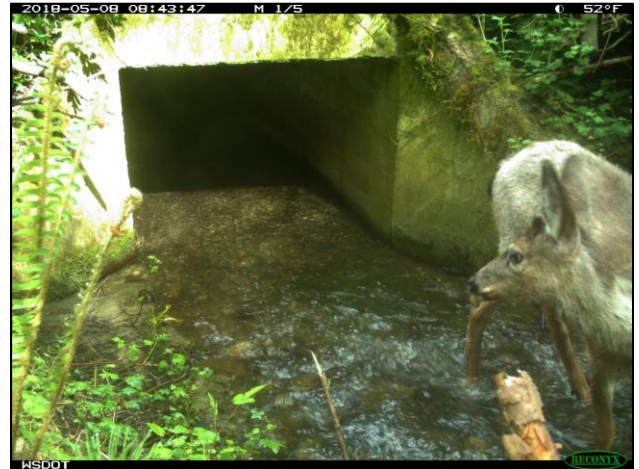
Figure 53. 990075 Before Construction: The old crossing was a concrete box culvert with a 3 ft span by 4 ft rise measuring 175 ft long and assessed as a barrier due to excessive water surface drop at the outlet.
