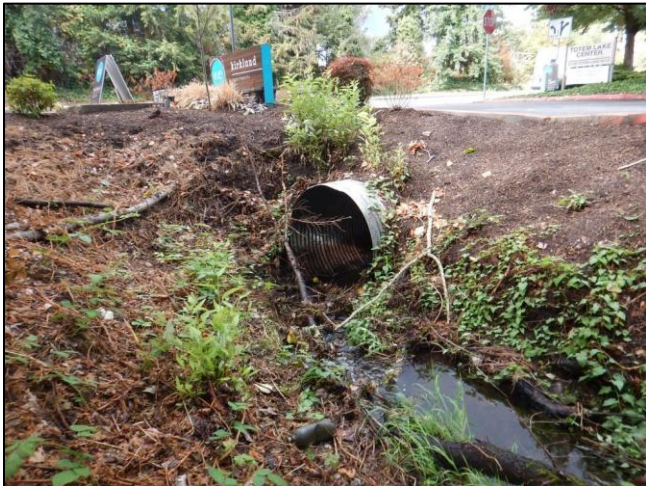
Figure 14. 992654 Before Construction: The old crossing was a single 4.5 ft diameter corrugated steel culvert with multiple catch basins. The approximate length of the structure was 843 ft and extended under 114 th Place NE, NE 132 nd St, all lanes of I-405 and Totem Lake Blvd NE. The culvert was a barrier to fish passage due to excessive slope.
