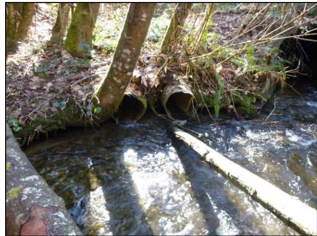
Figure 46. 933460 Before Construction: The old tributary crossing was a pair of 2 ft diameter corrugated steel culverts.
