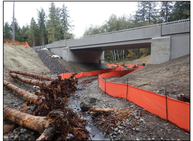
Figure 56. 990075 After Construction: The new crossing is a 55 ft span concrete bridge that facilitates passage for both fish and terrestrial wildlife.
