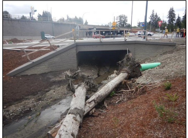
Figure 15. 992654 After Construction: The new structure is a bottomless arch culvert with a length of 174 ft. The culvert has a span of 18 ft and a rise of 6 ft. In addition to the culvert, the daylighted channel underneath the I-405 overpass runs a length of 255 ft.
