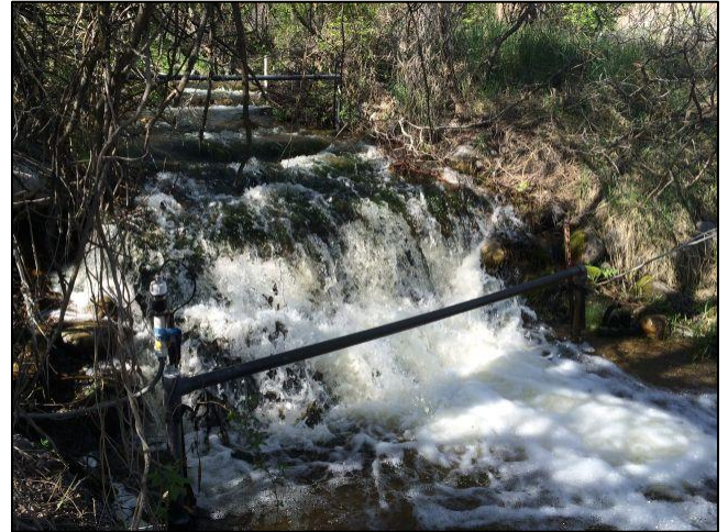
Figure 94. 960241 Before Construction: The upper of two dams located upstream of highway crossing removed during construction.
