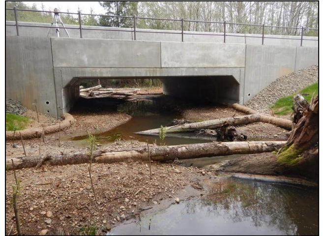
Figure 72. 991836 After Construction: The new crossing is a 26 ft span by 10.5 ft rise concrete box culvert.
