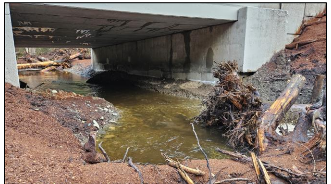
Figure 40. 997225 After Construction: Chum through the swimming upstream through the culvert.
