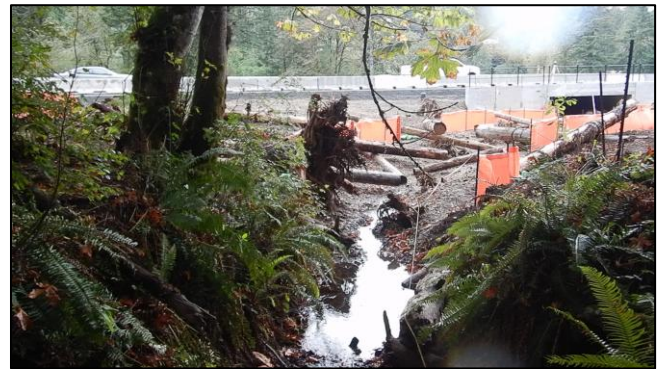
Figure 80. 990773 After Construction: The new crossing is an 18.17 ft span concrete box culvert.
