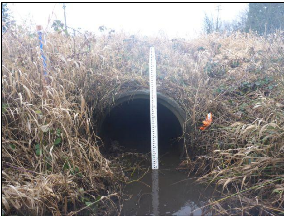
Figure 28. 935160 Before Construction: This crossing was originally a concrete culvert with a diameter of 3 ft. This culvert was 476 ft long and ran parallel to 70th Ave E and Barth Road.
