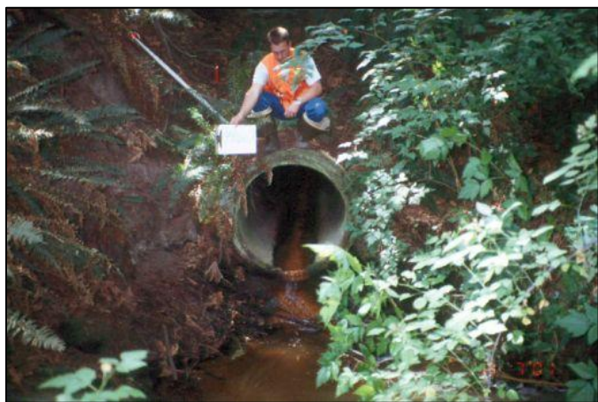
Figure 51. 991667 Before Construction: The old crossing was a 4 ft diameter corrugated steel culvert cobbled to a 3 ft diameter concrete culvert. The crossing was assessed as a barrier due to slope.
