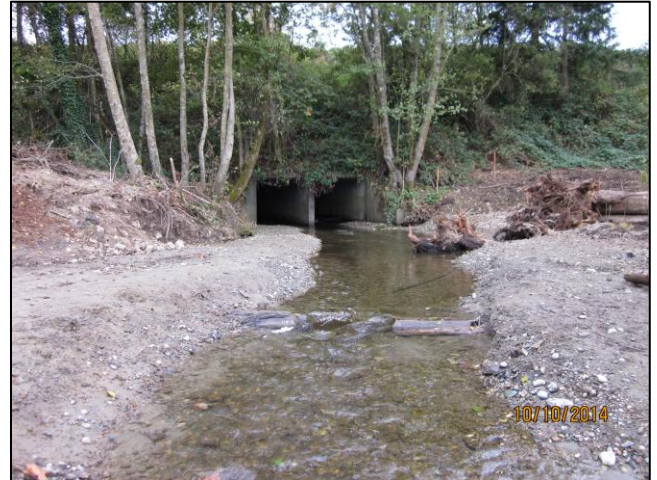
Figure 48. 15.0229 0.10 Before Construction: The old crossing was comprised of two concrete box culverts with a span and rise of 8 ft each and a length of 400 ft. In 2014, three baffles were installed inside one of the culverts and a single log weir was installed downstream of the outlet. Despite this effort to improve conditions, the site was determined to be a fish passage barrier in 2016.
