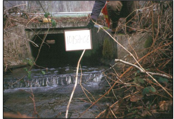
Figure 7. 101SA-06 Before Construction: The old crossing was 4 ft span by 2 ft rise concrete box culvert. It was a fish passage barrier due to excessive slope.
