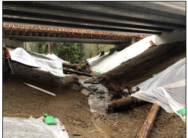
Figure 78. 993724 After Construction: The new crossings are two 84 ft-span concrete bridges on EB and WB SR 8.
