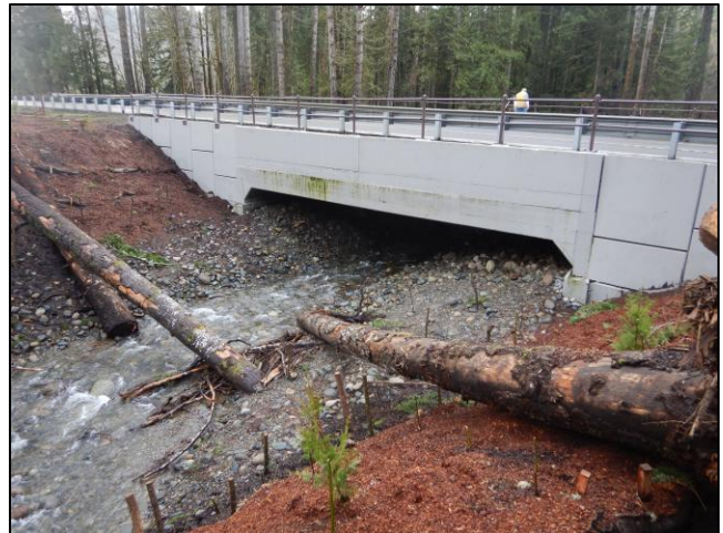
Figure 34. 991672 After Construction: The culvert was replaced with a 34.5 ft long bridge.
