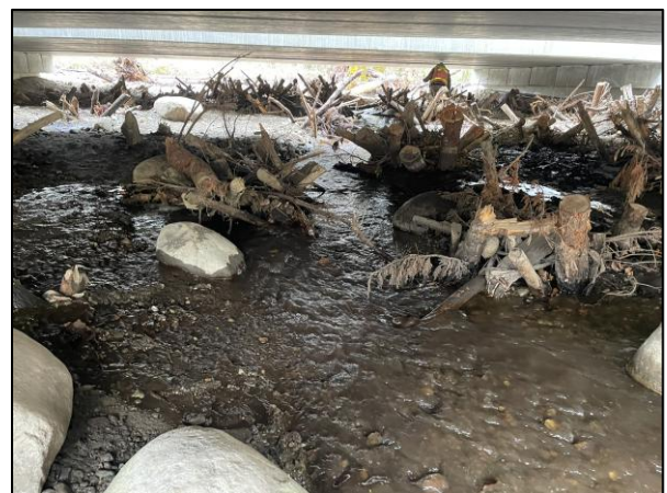
Figure 9. 101SA-06 After Construction: Slash cones under the new bridge.
