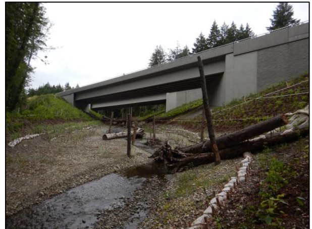
Figure 45. 15.0060 1.00 After Construction: The new crossing consists of two 198 ft long bridges for EB and WB traffic.
