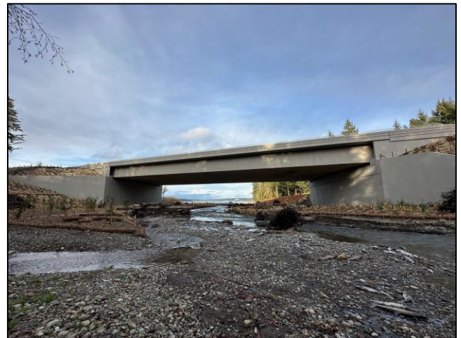
Figure 49. 15.0229 0.10 After Construction: The new crossing is a 205.5 ft long bridge that is located south of the original crossing. A section of the original upstream channel was regraded and incorporated into a small unnamed tributary that flows into the realigned mainstem, leading under the SR 3 bridge.
