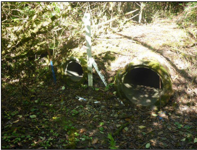
Figure 12. 932933 Before Construction: The old crossing consisted of two round concrete culverts. The first culvert had a diameter of 1.5 ft. The second culvert had a diameter of 2.5 ft. Each culvert was approximately 378 ft in length and extended under all lanes of I-405. Both culverts were barriers to fish passage due to excessive slopes.
