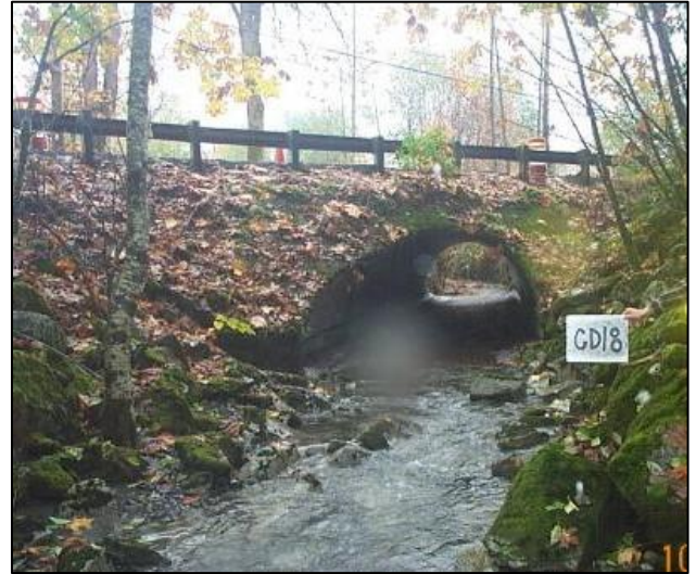
Figure 5. CD18 Before Construction: The old crossing was a 69 ft long squash structural plate steel culvert with 12.7 ft span by 8.3 ft rise. The crossing was assessed as a barrier due to excessive slope.
