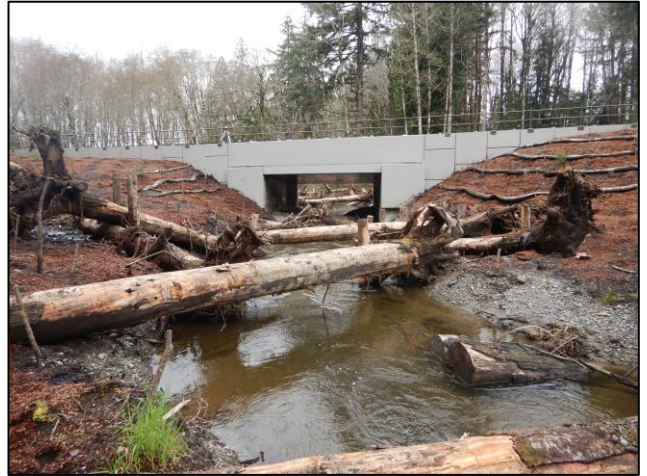
Figure 39. 997225 After Construction: The new structure is a 22.5 ft long concrete bridge.
