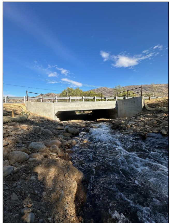
Figure 91. 990217 After Construction: The new crossing is a concrete bottomless arch culvert measuring 24 ft span, 9 ft rise and 91 ft long.
