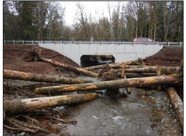
Figure 36. 990278 After Construction: The new structure is a concrete bottomless arch culvert with a span of 19 ft and a rise of 16.5 ft and is 47 ft long.
