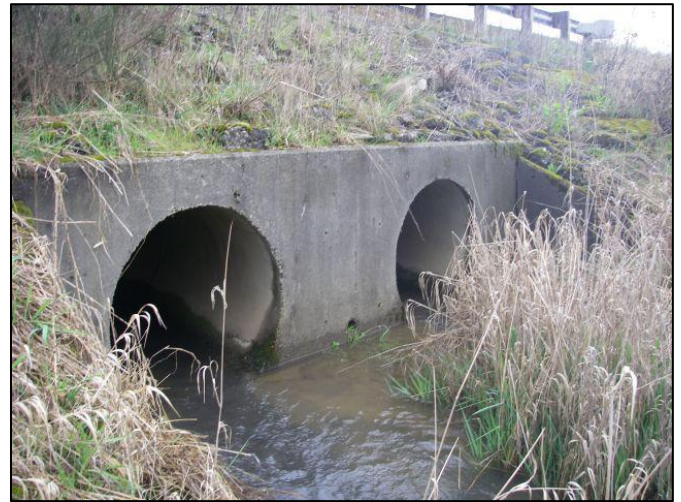
Figure 85. 125 1806W34G Before Construction: The old crossing was a double cell concrete culvert with each cell measuring 4 ft in diameter and 151 ft long. The old crossing was assessed as a depth barrier.
