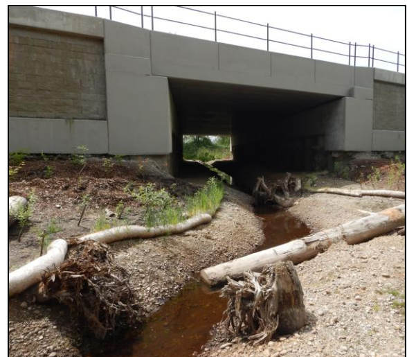
Figure 84. 933616 After Construction: The new crossing is a 26.5 ft span concrete bridge.
