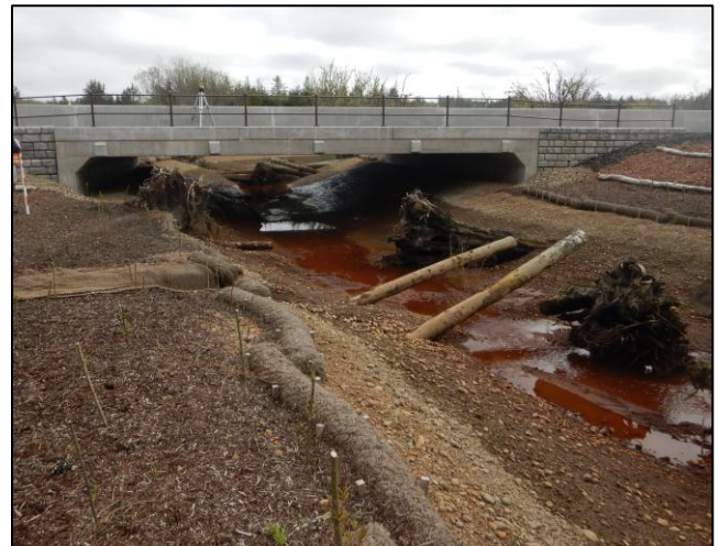
Figure 74. 990932 After Construction: The new crossing for 990932 is a 47 ft span by 14 ft rise concrete box culvert.
