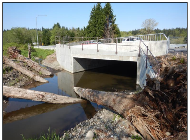
Figure 20. 996925 After Construction: The new crossing under SR 202 is a 25 ft span by 13 ft rise concrete box culvert.
