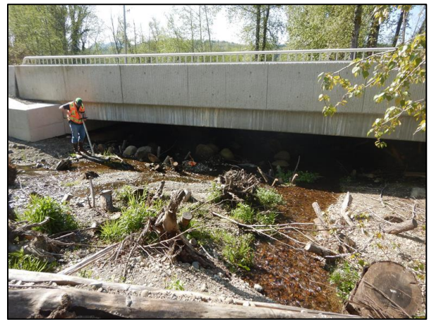
Figure 8. 101SA-06 After Construction: The new crossing is a 52 ft-span concrete bridge.
