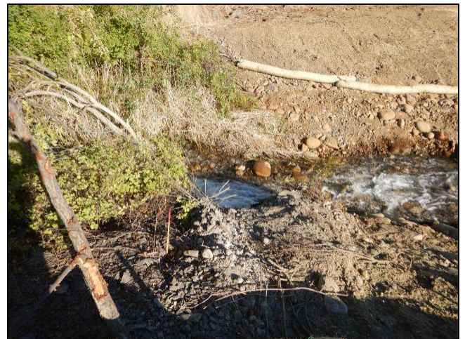
Figure 95. 960241 After Construction: The restored channel after dam removal to allow for fish passage.
