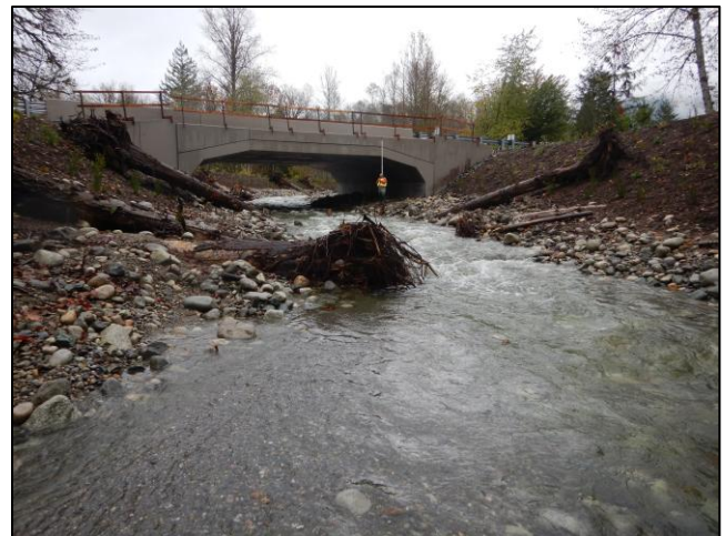
Figure 6. CD18 After Construction: The new crossing is a 40 ft span concrete bridge with wildlife benches lining each side of the channel.
