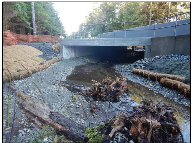
Figure 60. 997054 After Construction: The new crossing is a 23 ft span by 8 ft rise concrete box culvert.
