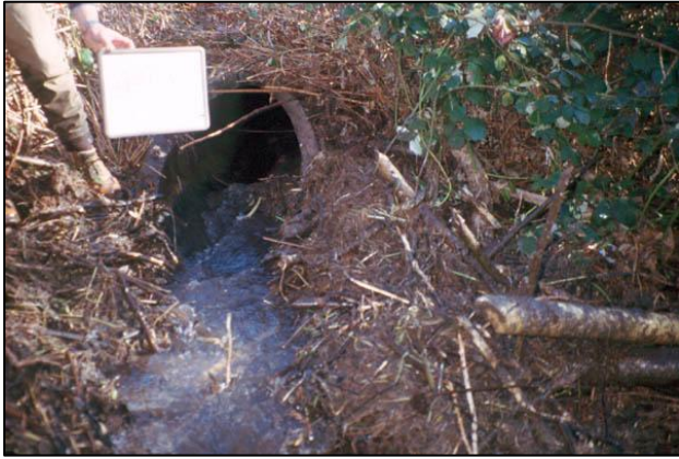
Figure 10. 995200 Before Construction: The old crossing was a culvert that crossed under both SR 202 and Fish Hatchery Road. It was a round concrete culvert with a diameter of 2 ft and was a fish passage barrier due to excessive slope.
