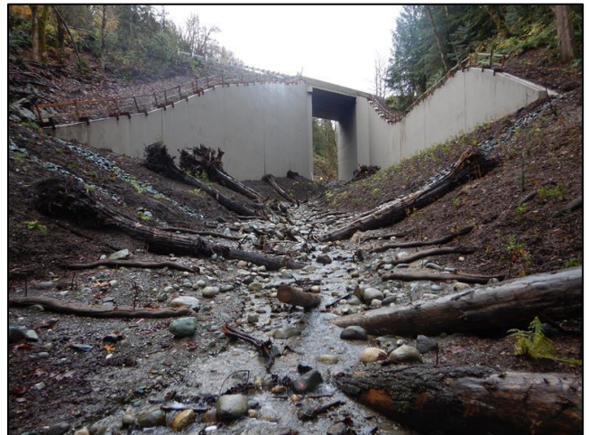
Figure 4. 991126 After Construction: The new crossing is a 29 ft clear span concrete bridge.
