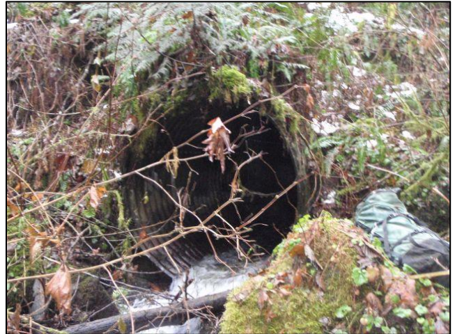
Figure 3. 991126 Before Construction: The old crossing was a 5.74 ft round steel plated culvert measuring 322 feet long. The culvert was assessed as a barrier due to excessive water surface drop at the outlet.
