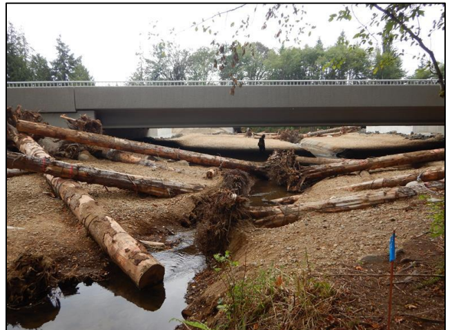
Figure 82. 22.0349 0.70 After Construction: The new crossings are 106 ft span concrete bridges.
