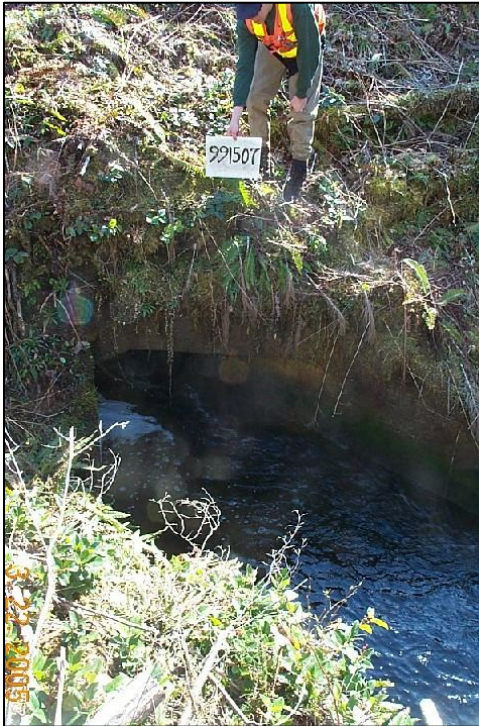
Figure 63. 991507 Before Construction: The old crossing was a 4 ft diameter concrete culvert cobbled to a 4 ft span by 3 ft concrete box culvert and was a barrier due to slope.
