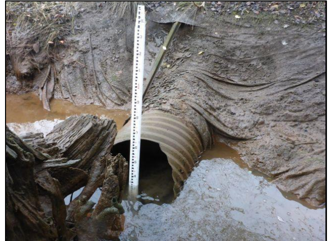
Figure 73. 990932 Before Construction: The old crossing for SR 109 was a 2 ft diameter corrugated steel culvert with a log control fishway to facilitate passage.
