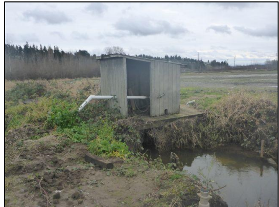
Figure 26. 935159 Before Construction: This crossing was a single span bridge constructed with wood planks. An abandoned pumphouse was located on the structure. During the previous site assessment, it was determined that this site was not a barrier to fish passage.
