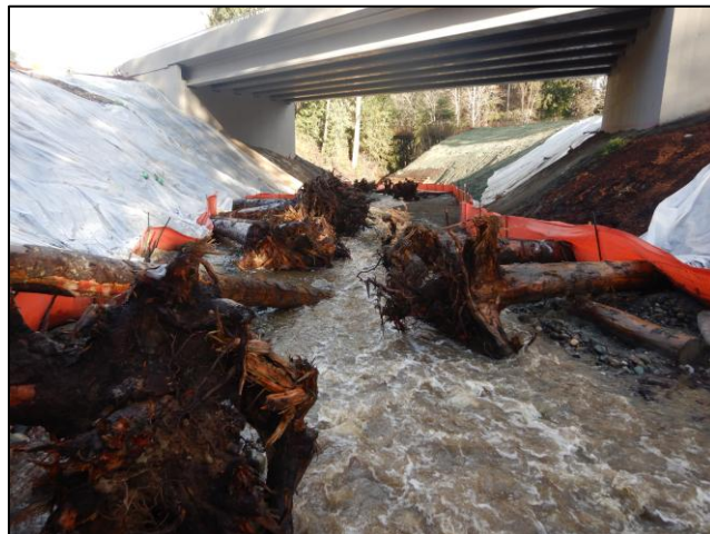
Figure 52. 991667 After Construction: The new crossing is a 116 ft long concrete bridge.
