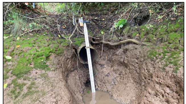
Figure 75. 935978 Before Construction: The old WSDOT mitigation area driveway crossing was a 2 ft diameter corrugated steel culvert.
