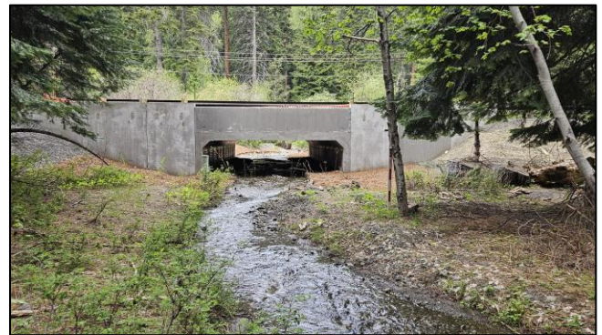
Figure 89. 998490 After Construction: The new crossing is an 18 ft span, 8 ft rise precast concrete box culvert. The new channel has a short tie-in. Large wood was not installed because the focus of the project was to allow unimpeded sediment transport through the crossing. Type 2 boulders were placed in the interior to prevent entrainment in the event of scour.
