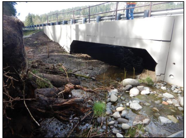
Figure 43. 936719 After Construction: The new structure for the SB lanes (936719) is a 19 ft span by 12.5 ft rise bottomless arch culvert and was assigned a new Site ID.
