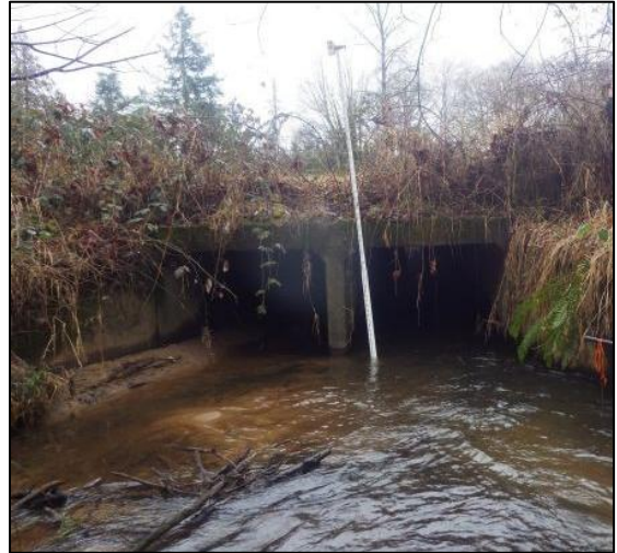
Figure 81. 22.0349 0.70 Before Construction: The old crossing was a double cell concrete box culvert with each cell measuring 6 ft span by 6 ft rise and 273 ft long under 10 ft of road fill. Two downstream fishways associated with the crossing, previously installed as streambed controls, were nonfunctioning and were consequently removed.
