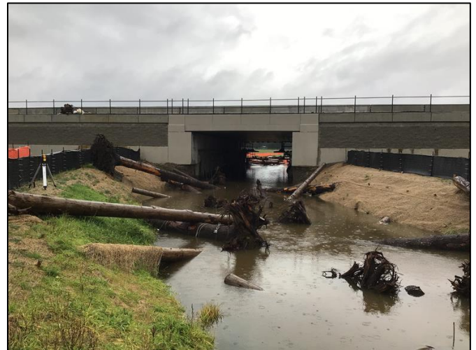
Figure 86. 125 1806W34G After Construction: The new crossing is a 26 ft span concrete bridge.
