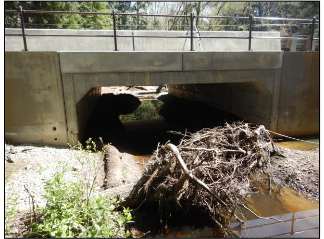
Figure 66. 990920 After Construction: The new crossing is a 19 ft span by 11 ft rise concrete box culvert.
