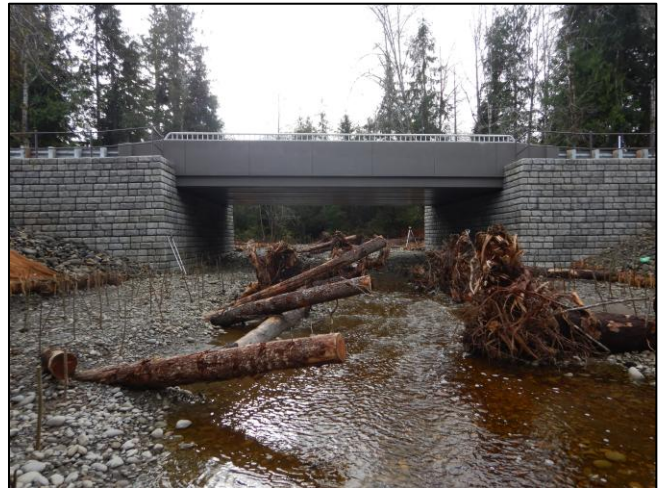
Figure 62. 991575 After Construction: The new crossing is a 42 ft long concrete bridge.
