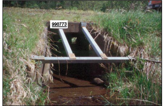
Figure 79. 990773 Before Construction: The old crossing was 4 ft span by 4 ft rise concrete box culvert measuring 140 ft long. The structure was a barrier due to water velocity.
