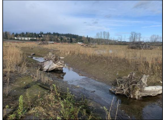
Figure 25. 935158 After Construction: The crossing was removed and channel realigned. The location of the original crossing is now associated with one of many side channels along the new stream alignment.
