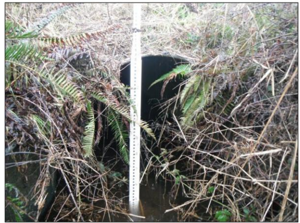
Figure 83. 933616 Before Construction: The old crossing consisted of two round corrugated steel culverts. Both 4.5 ft diameter and measuring approximately 167 ft long. The site was assessed as a barrier due to water depth.
