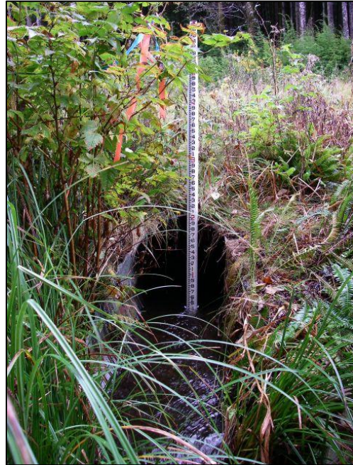
Figure 59. 997054 Before Construction: The old crossing was a 2 ft diameter steel culvert and was a barrier due to velocity.
