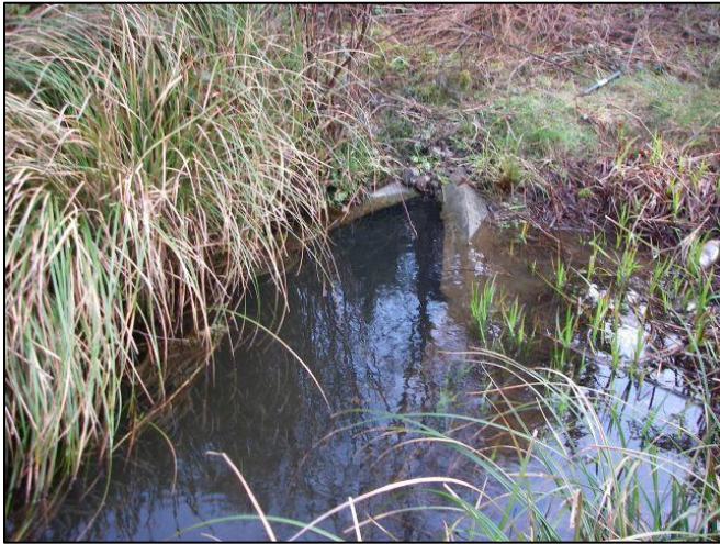
Figure 71. 991836 Before Construction: The old crossing was a 3 ft diameter concrete culvert and was a barrier due to velocity.
