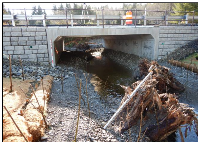
Figure 58. 990717 After Construction: The new crossing is a 20 ft span by 12 ft rise concrete box culvert.
