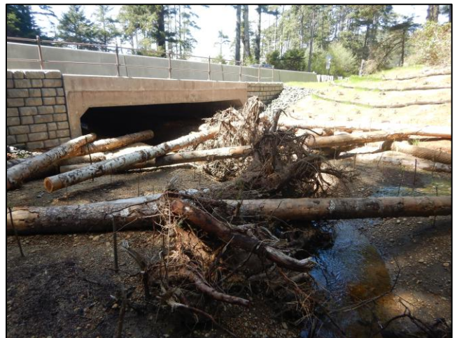
Figure 68. 997363 After Construction: The new crossing is a 26 ft span by 10 ft rise concrete box culvert.
