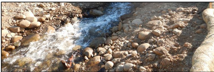
Figure 93. 960240 After Construction: With barrier now removed, the newly constructed downstream channel enables fish passage.
