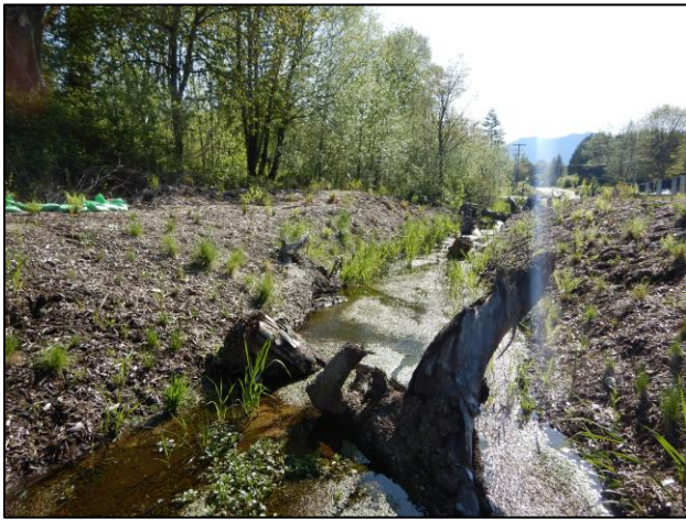
Figure 11. 995200 After Construction: This site is now an open channel with no road crossing.
