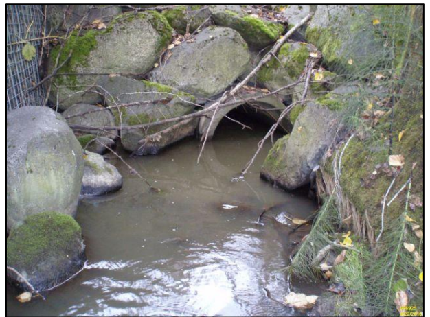
Figure 19. 996925 Before Construction: The old crossing was a 3 ft diameter concrete culvert. This structure was a fish passage barrier due to excessive slope.
