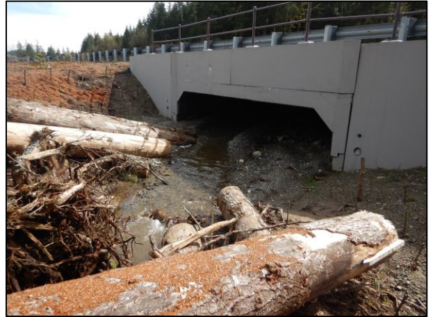
Figure 42. 997161 After Construction: The project replaced the single culvert with two separate structures for NB and SB lanes. The new structure for the NB lanes (997161) is a 19 ft span by 13 ft rise bottomless arch culvert.
