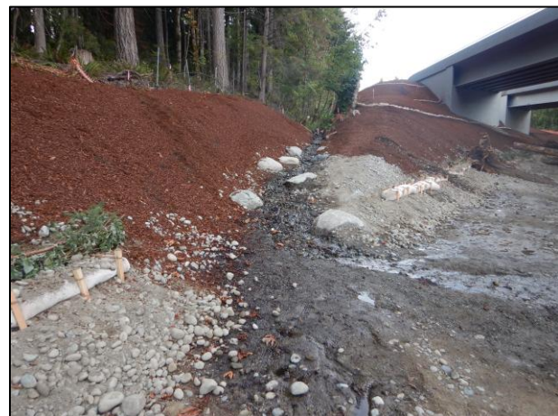
Figure 47. 933460 After Construction: The abandoned tributary crossing is now open channel.
