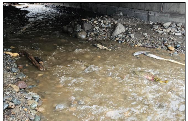
Figure 37. 990278 After Construction: Over the winter following installation, adult chum were observed spawning throughout the project area.
