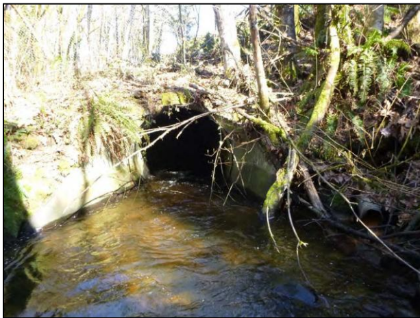
Figure 44. 15.0060 1.00 Before Construction: The old crossing was 6 ft diameter metal culvert retrofitted with a fishway and was a barrier to chum, coho, steelhead, coastal and resident trout. The culvert was 544 ft long and was a barrier due to velocity.
