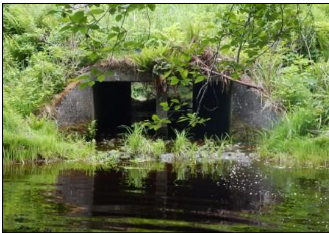
Figure 61. 991575 Before Construction: The old crossing was a 2-cell concrete box culvert with each cell measuring 5 ft span by 5 ft rise and was a barrier due to slope.
