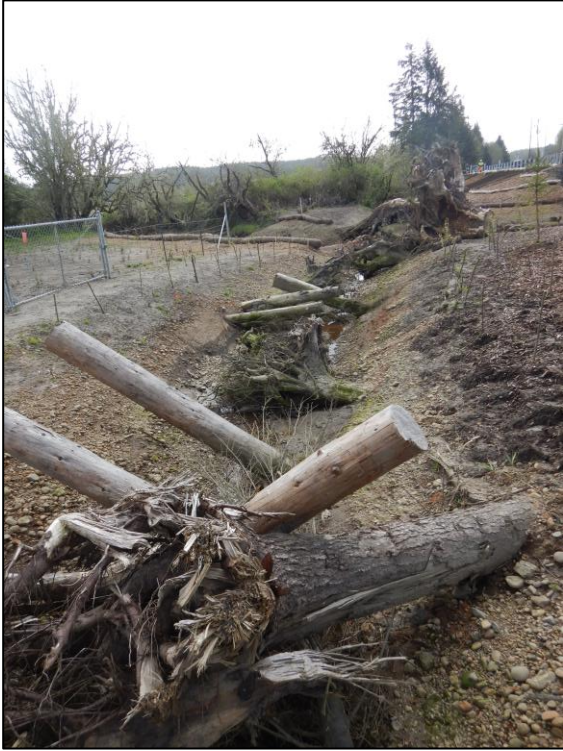
Figure 76. 935978 After Construction: The open channel.
