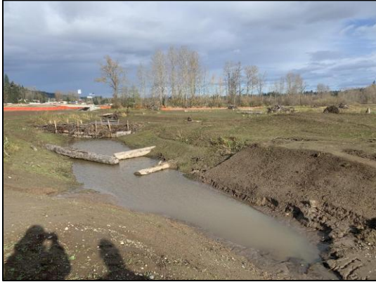
Figure 23. 935157 After Construction: The crossing was removed and channel realigned. The location of the original crossing is now associated with a backwatered side channel along the new stream alignment.
