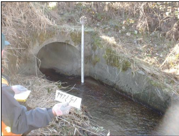
Figure 41. 997161 Before Construction: The old crossing was a 3 ft diameter concrete culvert that extended under all lanes of US 101 and was a barrier to fish passage due to slope.
