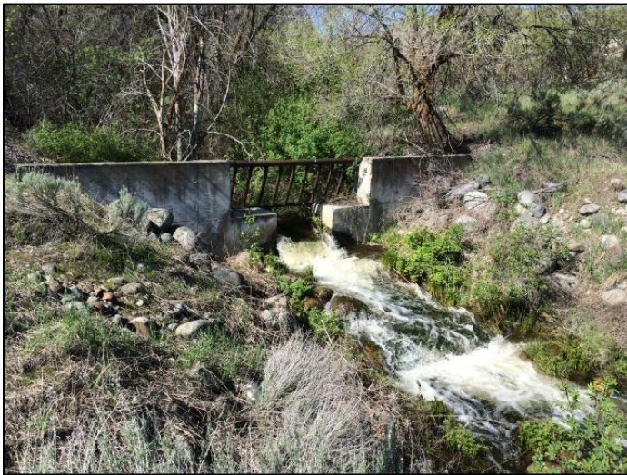
Figure 92. 960240 Before Construction: Although not a motorized crossing, it was the lower of two dams located immediately upstream of WSDOT US 97 crossing. It was one of two remnants of the old diversion system used to exclude debris.
