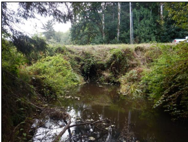
Figure 38. 997225 Before Construction: The old crossing was a 72 ft long, 5 ft diameter structural plate steel culvert. The crossing was assessed as a fish barrier due to both low flow depth and high flow velocity.
