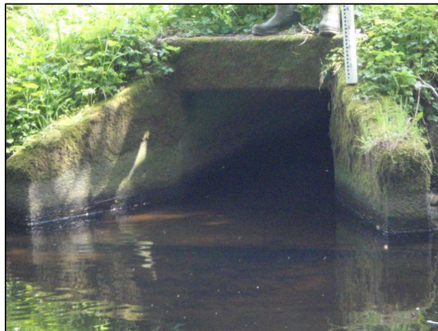
Figure 57. 990717 Before Construction: The old crossing was a 3 ft span by 3 ft rise concrete box culvert and was a barrier due to slope.
