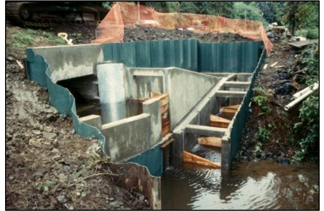
Figure 35. 990278 Before Construction: The old crossing was a 6 ft by 4 ft concrete box culvert and was retrofitted with a 9 weir-pool fish ladder to improve access upstream for migrating salmonids. Due to continued and chronic aggradation, the ladder was deemed ineffective at providing fish passage in 2015.
