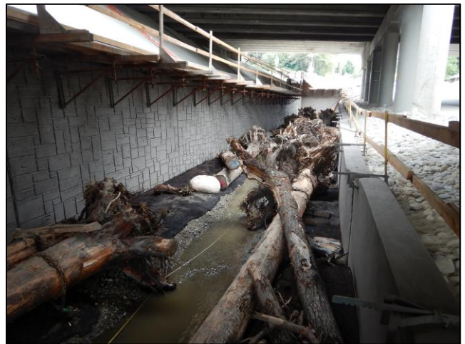
Figure 16. 936700 After Construction: Site 936700 is a daylighted section of channel that flows along NE 132 nd St underneath the I-405 overpass directly upstream of the new WSDOT structure for the southbound off ramp. This section is walled along both banks and contains several LWM structures to add complexity to the stream.
