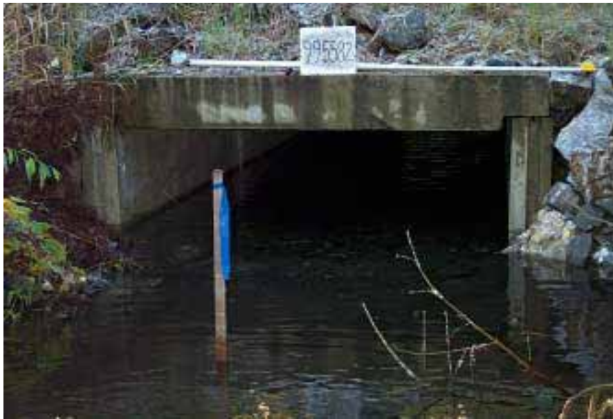
Figure 39. As part of the 2004 and 2005 WSDOT highway improvement project, numerous undersized culverts were replaced with larger ones, improving fish passage and drainage during spring snow melt. This 2.45 m wide concrete box culvert benefits resident trout.
