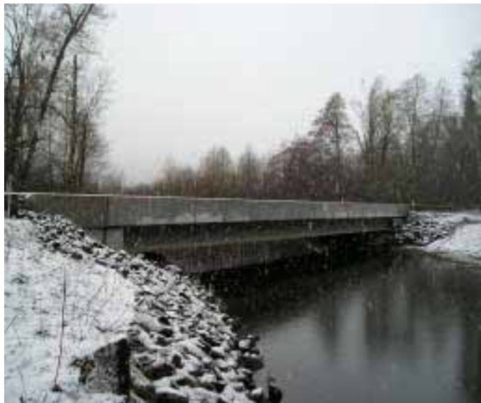
Figure 11. In 2005, WSDOT replaced the box culvert with a 37 m wide single span bridge through a Dedicated Funding (I-4) project. The new bridge provides an unlimited access to over 4.5 acres rearing habitat to coho and chinook salmon, steelhead, resident and searun cutthroat trout, as well as restores the channel and improves creek flow capacity under the highway during storm events. The construction cost of this $1.8 million bridge was a multi-agency effort involving the Hood Canal Salmon Enhancement Group, Skokomish Tribe, and WSDOT.
