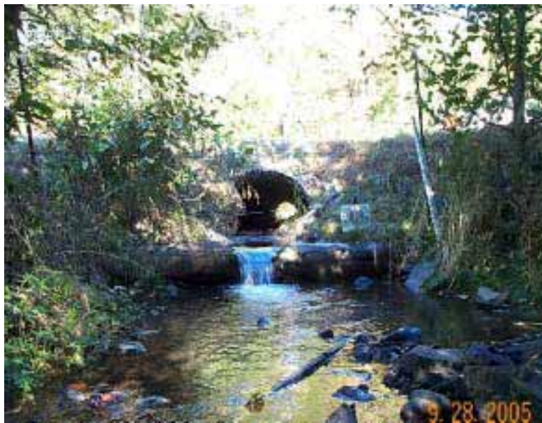
Figure 41. Eight log controls were placed downstream of a squash, corrugated steel, 1.65 m wide culvert to backwater the culvert and improve access to 900 meters of habitat for resident trout.
