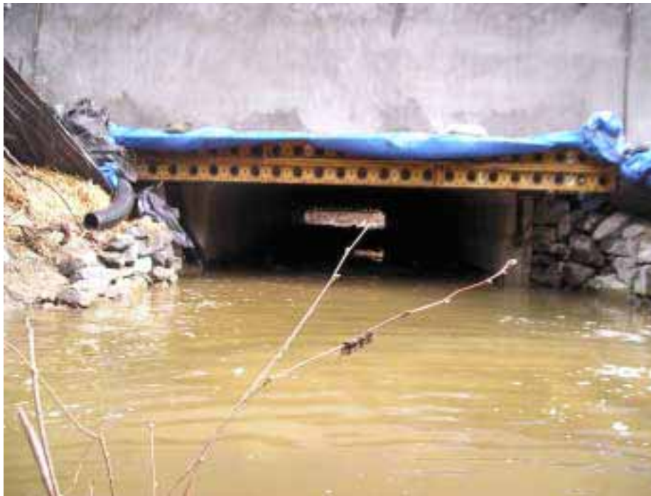
Figure 28. Installed in 2005, the new, larger concrete, 3.7 m wide box culvert with natural streambed material throughout will provide unimpeded fish passage to over 3,000 meters of potential habitat for coho salmon, steelhead and resident trout. In addition to providing fish passage, the new culvert will be able to accommodate 100 year flows, and reduce erosion.
