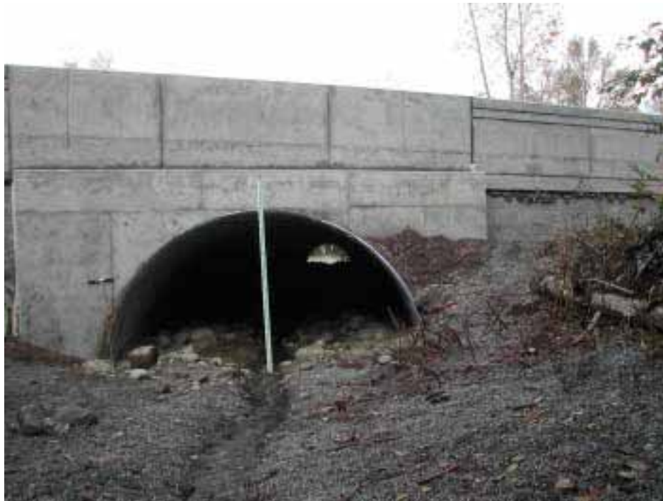
Figure 31. A 4.10 m wide structural plate steel arch culvert was installed in 2005 replacing the under-sized culvert. The new culvert is set at a slope of less than 1% and has natural streambed material throughout, providing unobstructed fish passage to over 2,700 meters of habitat for coho salmon, steelhead, resident, and searun cutthroat trout.
