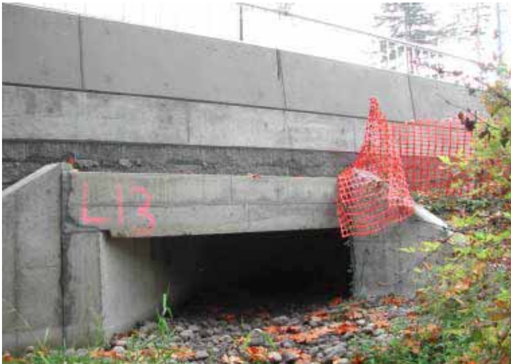
Figure 36. WSDOT replaced a 1.2 m wide, concrete box culvert with a 2.4 m wide, concrete box culvert, improving fish access to 37 acres of rearing habitat at the same time increasing creek flow capacity under the highway during extreme flows. The new culvert was a part of a 2005 Safety and Mobility project, where WSDOT widened the existing two-lane road to a four-lane one, replaced undersized culverts, and improved water quality through the construction of new detention ponds.
