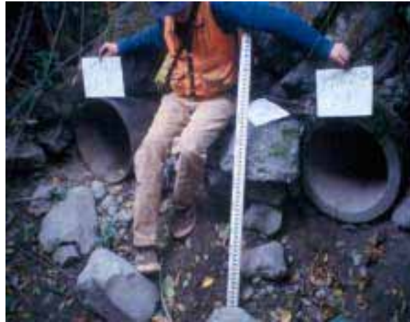
Figure 27. Two .46 m wide steel and concrete (left and right) pipes were considered barriers due to a slope of 1.8% and 2.1% respectively.
