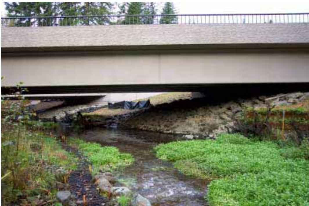
Figure 19. A full-span bridge was constructed in 2005 during the SR 18 Safety and Mobility project. Coho salmon, steelhead and resident trout can fully utilize over 1,600 meters of habitat above the new bridge.
