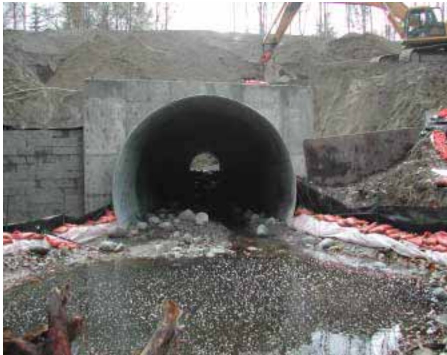
Figure 34. A 4.10 m wide corrugated steel culvert was installed in place of the old pipe in 2005 during a road widening project. Coho salmon, steelhead and resident trout will benefit from 370 meters of potential rearing habitat upstream of this crossing.
