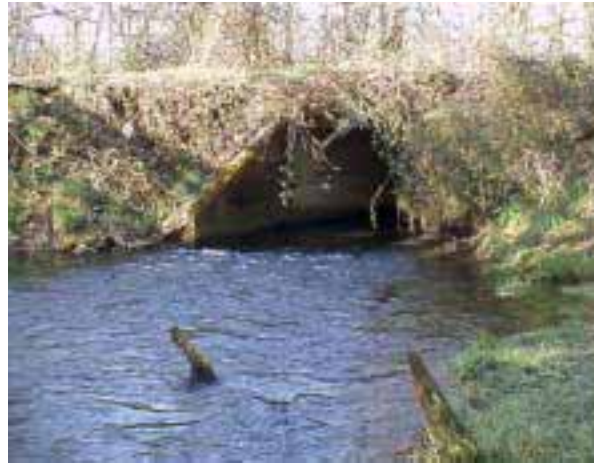
Figure 10. A 1.83 m wide, concrete box culvert was identified as a barrier due to excessive water velocity evidenced by bank scouring downstream of the culvert.
