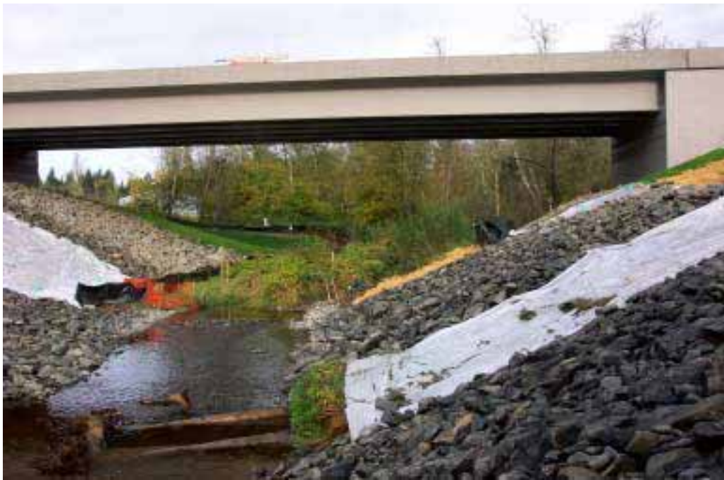
Figure 19. A new bridge was constructed in 2005, during the SR 18 highway improvement project involving the construction of a 4 four-lane divided highway. WSDOT replaced seven culverts in Taylor Creek and its tributaries with full-span bridges between 2003 and 2005 at a cost of $9.72 million. The cost of this bridge was $2.14 million. Over 3,300 meters of potential habitat for coho salmon, steelhead and resident trout is now easily accessible. Another SR 18 culvert upstream of this crossing was replaced with a bridge in 2005 as well (See Figures 21 and 22).
