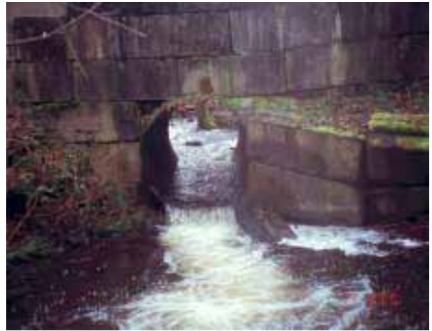
Figure 24. The original 1.8 m round steel culvert was equipped with downstream rock controls. The rock controls were not effective in backwatering the culvert and the outfall drop gradually increased to 0.27 m obstructing fish passage.
