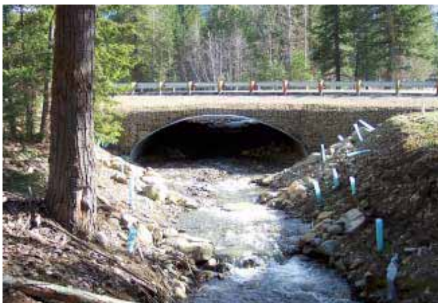
Figure 14. In 2005, the steel culvert was replaced with an 8 m wide structural plate steel arch stream simulation culvert allowing unrestricted fish access to over 5,000 meters of upstream habitat. In addition to restoring fish passage for chinook salmon, steelhead, bull trout and resident trout, the Dedicated Funding (I-4), $545,000 project alleviated maintenance issues associated with clearing debris caught inside the baffled culvert and increased the culvert's capacity to accommodate 100 year flood flows.
