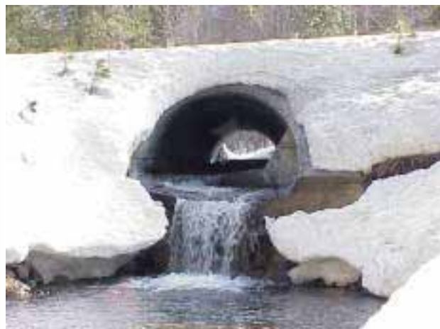
Figure 13. A 1.85 m high outfall drop on the downstream end of a 2.72 m wide structural steel plate culvert created a fish passage barrier to chinook salmon, steelhead, bull trout and resident cutthroat trout. The culvert was equipped with 13 baffles, which required frequent maintenance.
