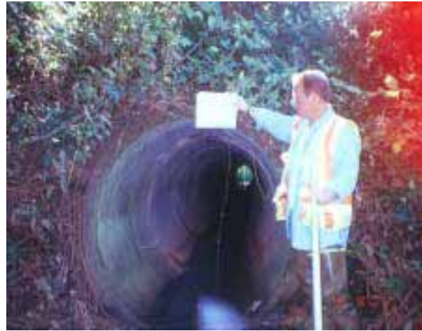
Figure 21. A round, 1.52 m concrete culvert was considered a barrier due to a 2.25% slope.
