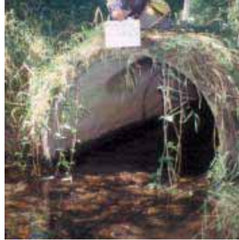
Figure 18. A round, 1.52 m wide concrete culvert was undersized.
