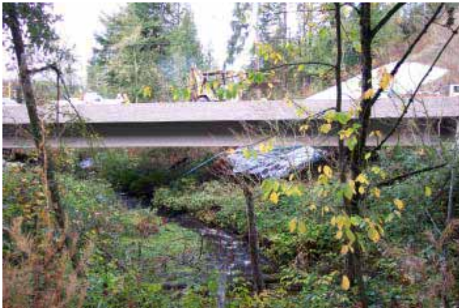
Figure 25. Fish passage at this crossing was addressed in 2005 during the SR 18 widening project. WSDOT replaced the old steel culvert with a full span bridge for a total cost of $291,600. The new bridge improved fish access to 7,400 meters of potential habitat upstream for coho salmon and resident cutthroat trout.
