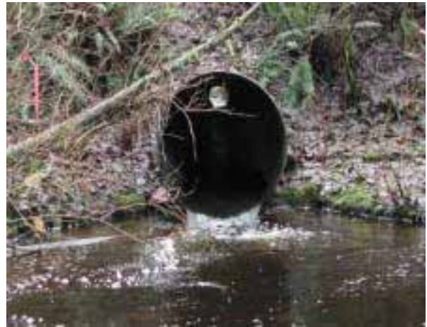
Figure 30. A 1.2 m wide, round corrugated steel culvert was a velocity barrier.
