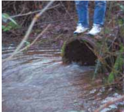
Figure 33. A .61 m wide concrete culvert was a barrier to fish passage due to 2% slope.
