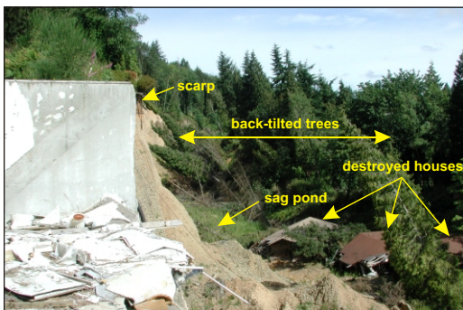
Figure 1. View northwest along the main scarp of the Aldercrest-Banyon landslide (1998) as it appeared in August of 2000. Note the destroyed houses and tilting trees at the base of the scarp. Prior to the landslide, these houses were slightly above the elevation of the top of the scarp. This photo was taken in the former basement (light gray area on the left) of a house now at the bottom of the hill outside the photo area. The scarp exposes Neogene fluvial gravels and sands of the Troutdale Formation.
