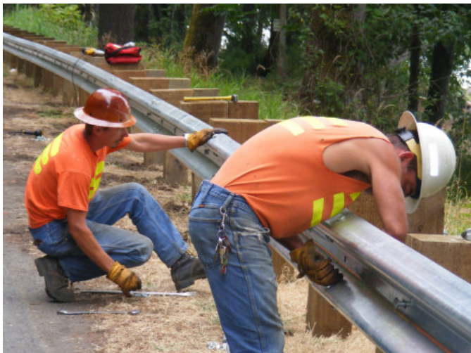
Workers for Pacific Rim Service & Construction Co. install guardrail along SR 4 in southwest Washington.
