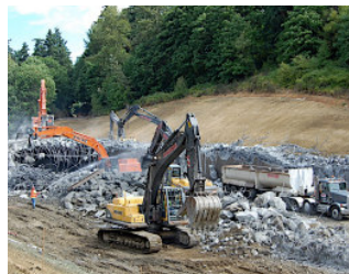
A worker is dwarfed by giant demolition equipment removing the Wilburton Tunnel in 2008.
