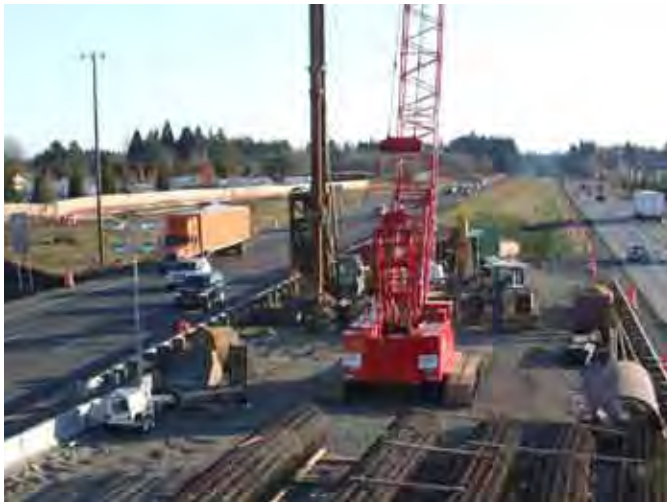
Crews are drilling in the I-5 median where the support column for the new SR 501 bridge will go.
