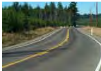
Example of chip seal roadway surface.
