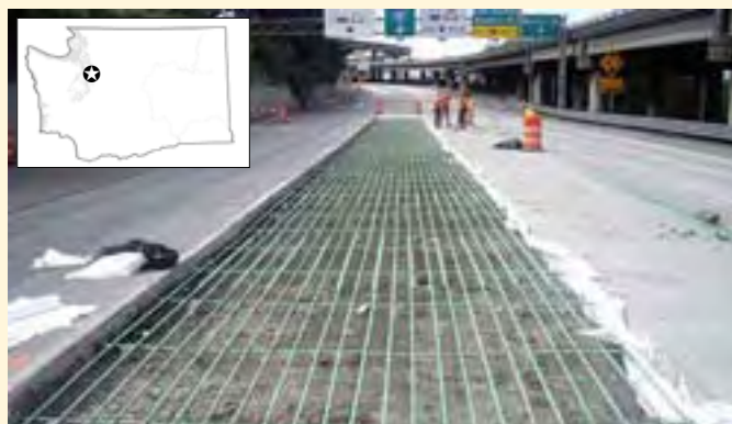
This project repaired and replaced about 440 concrete panels on I-5 in King County.
