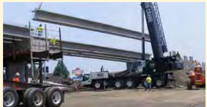
New, 110-foot-long girders are set on the new 112th Connector bridge during construction in June 2009.
