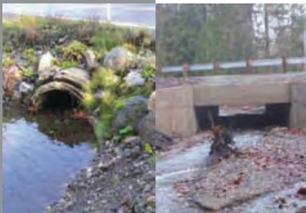
Before and After pictures of a barrier correction on SR 532 over Bruce Creek near Maple Falls. The 4-foot round culvert (left) was replaced with a 15-foot wide box culvert (right)
