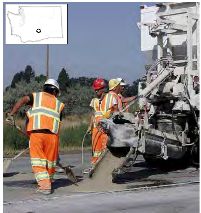
Granite NW Inc. crews place concrete over dowel bar slots on I-82 near Sunnyside.
