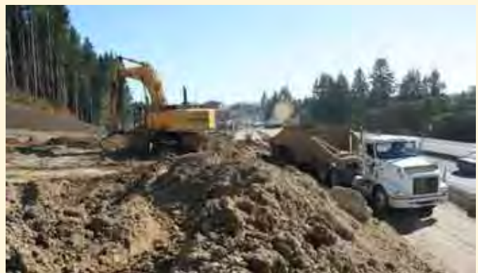
Above: The excavation site along I-5 near Grand Mound was affectionately deemed 'The Big Cut' by the construction crew because of the amount of dirt that was removed from the site.
