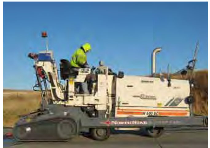
Crews are using this machine on US 195 near Colfax to cut rumble strips into the highway centerline. About 3 to 4 miles can be completed per day.
