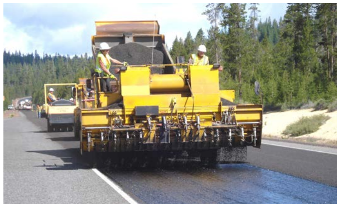
Resurfacing asphalt roadways with chip seal pavement saves WSDOT approximately $12,000 per year for every lane mile converted.
