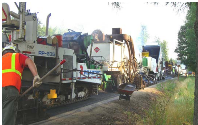
Hot-in-place asphalt paving (shown above on State Route 542 near Deming) requires a long train of equipment to heat, loosen, remove, reconstitute and repave the asphalt in one pass.
