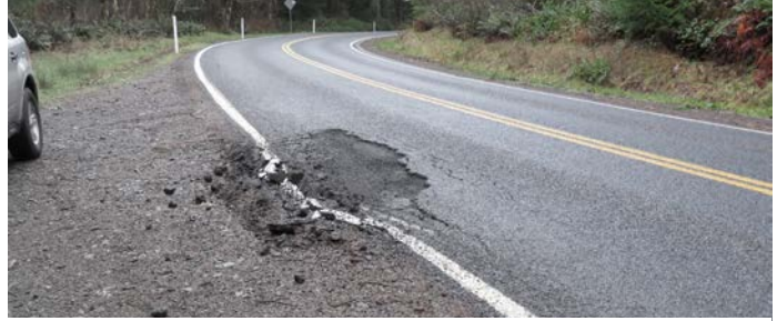
Several sections of State Route 100 near Ilwaco were damaged in 2014 by heavy truck traffic. As a result, WSDOT reduced the speed limit from 35 mph to 25 mph to help reduce further deterioration of the roadway.
