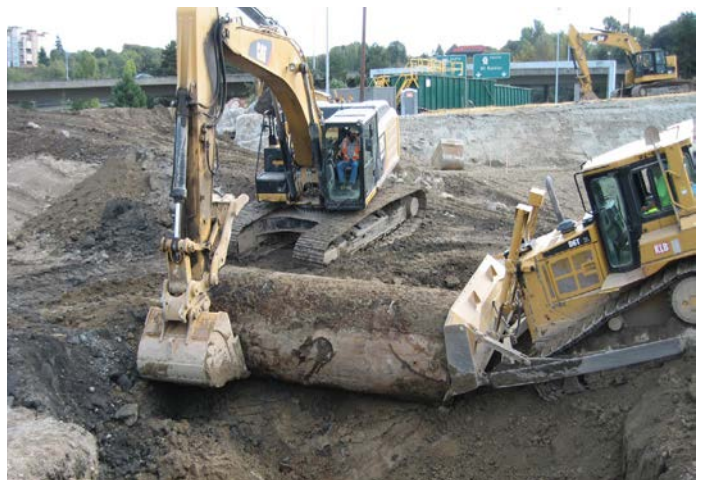
WSDOT's contractors improve the environment by removing old underground storage tanks on the Interstate 5 – M Street to Portland Avenue Project in Tacoma.
