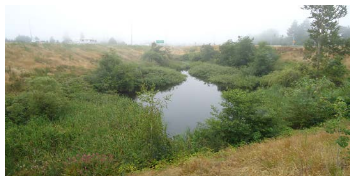
This stormwater basin has overgrown vegetation and does not adequately filter sediment from stormwater runoff. Approximately 19 percent of WSDOT's stormwater facilities are not yet in compliance.
