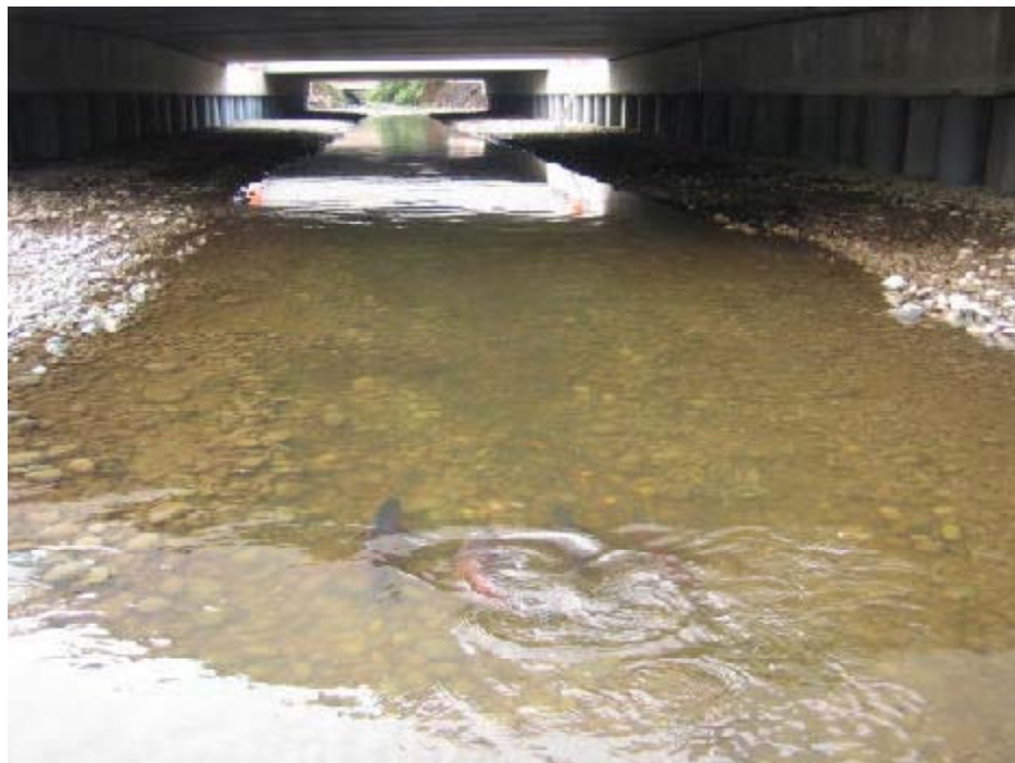
Figure 19. A new 24 m wide and 15 m long bridge was constructed in 2004, during a road improvement project. The construction cost of the Tibbetts Creek bridge was $4.3 million and the design cost $ 1 million. Coho salmon are seen spawning under the newly constructed bridge. Tibbetts Creek offers 9,400 m of potential habitat for coho and sockeye salmon, steelhead and resident trout. No known fish passage barriers exist downstream, however, 5 fish passage barriers including 4 WSDOT barriers located on SR 900 were identified upstream of the new bridge.
