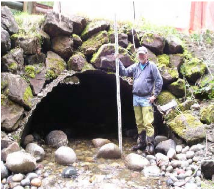
Figure 29. Upstream end of the culvert. Large rocks positioned inside the culvert effectively retain natural streambed material.
