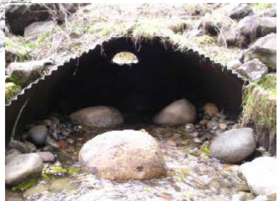
Figure 29. Upstream end of the culvert. Large rocks positioned inside the culvert effectively retain natural streambed material.
