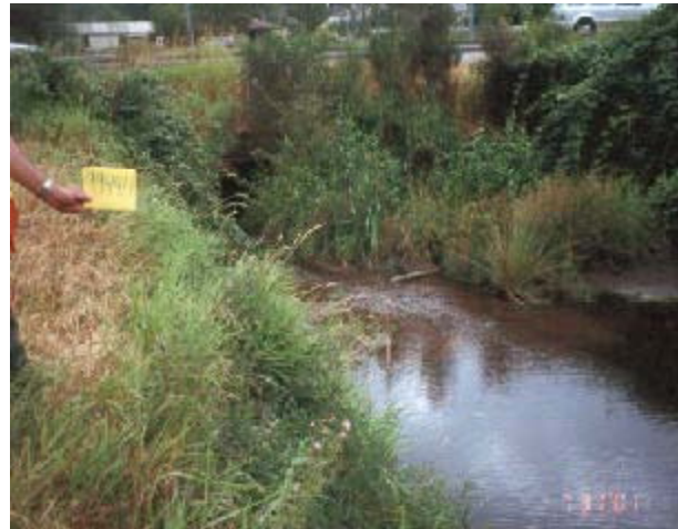
Figure 18. Three round, 1.22 m wide steel culverts were considered barriers due to a slope of 1.05 %.
