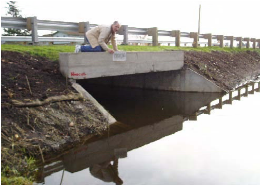
Figure 25. In 2004 WSDOT addressed road maintenance and fish passage issues by installing a new 4.4 m wide concrete box culvert. The $192,000 project improved fish access to 13,700 m of the potential habitat upstream for chum and coho salmon, steelhead, searun and resident cutthroat trout. Five culverts identified upstream need further barrier status assessment. There are at least two additional barriers downstream of the new WSDOT crossing.
