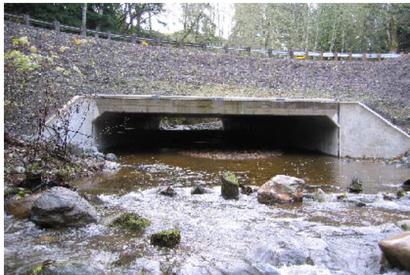
Figure 11. A large, 8.5 m wide and 44 m long bottomless precast concrete arch culvert replaced the old steel pipe. The construction of the culvert including excavation of 8 m of road fill cost $870,000. The culvert bottom simulates the natural conditions of the creek bed. The new culvert opened 11,500 m of stream habitat for chum and coho salmon, steelhead, resident and searun cutthroat trout. Two privately owned barriers exist upstream of the WSDOT crossing, blocking access to 2,600 m of additional habitat. One privately owned partial barrier remains downstream, at the mouth of Jim Creek.
