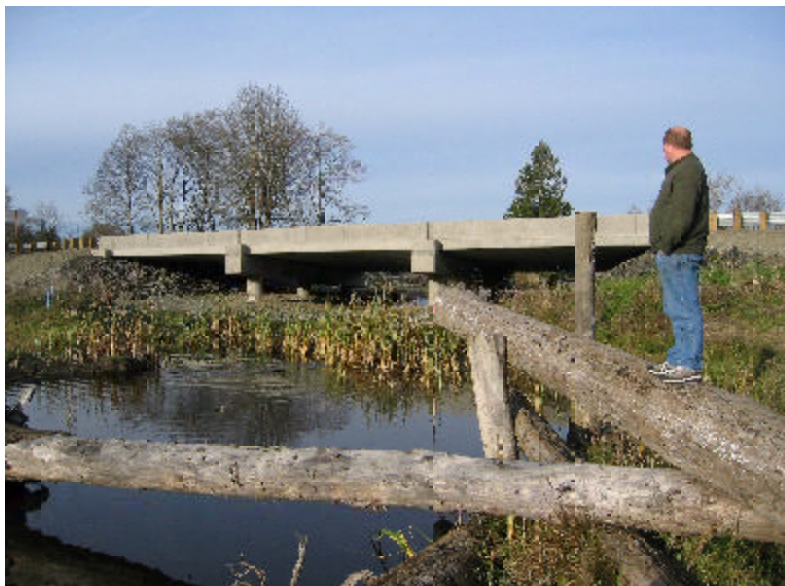
Figure 14. In 2004, the old double box culvert was replaced with a new, 30 m wide bridge. Construction of the new bridge marked the culmination point of a multi-entity effort involving the construction of a new channel and extensive habitat restoration upstream and downstream of the culvert. The $1.3 million project opened 10,000 m of habitat to chum and coho salmon, steelhead, searun and resident cutthroat trout. No known barriers exist downstream or upstream of the new bridge.
