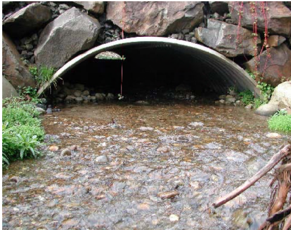
Figure 22. A 3.5 m wide, structural plate, arch culvert was constructed in 2004 by the Hood Canal Salmon Enhancement Group and a private developer. The downstream and upstream invert have been countersunk 50% below the streambed. The new culvert improved fish access to an estimated 1,000 m of habitat upstream for searun and resident cutthroat trout. At least one, privately owned barrier culvert exists downstream of this culvert. There are no known fish passage barriers upstream.
