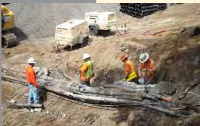
Utility crews work on lowering phone and cable lines below the construction work near I-205 in Clark County
