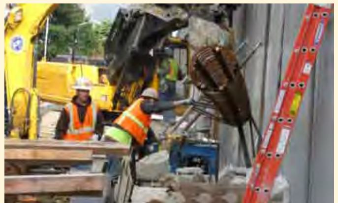
A steel cage is used for the foundation of the new noise wall. Crews position the cage in place over the foundation
