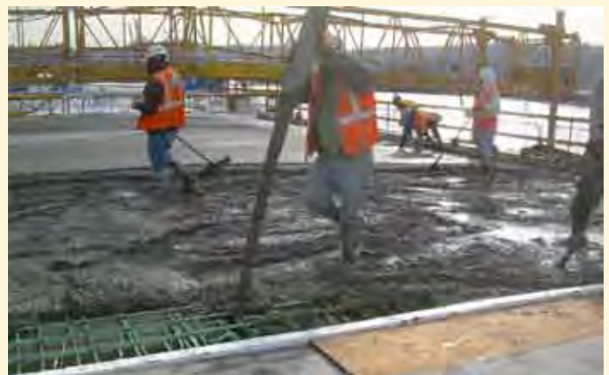
Structural concrete being poured on the new bridge deck of the SR 104 Hood Canal Bridge in May, 2009.
