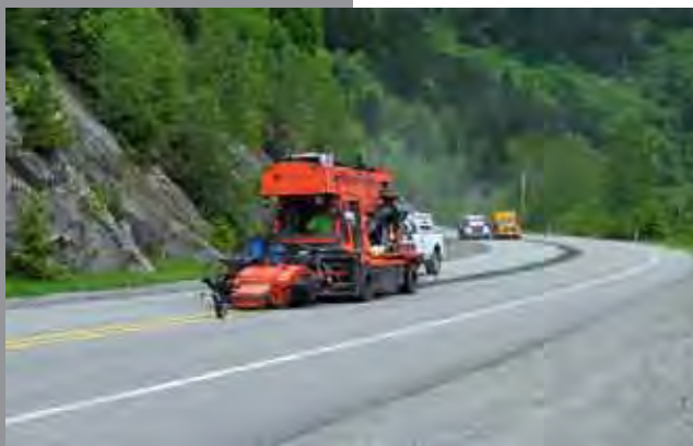
Crews ground 30 miles of centerline rumble strips on US 2 between Gold Bar and Stevens Pass in June 2008. The centerline rumble strips are an example of low-cost, near-term solutions that reduce collisions.
