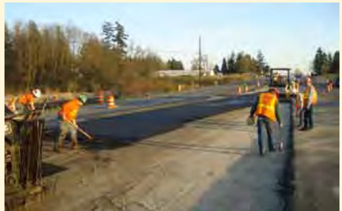
A hot mix asphalt (HMA) pour on the SR 539 Ten Mile Road project in April, 2009. HMA accounts for nearly half of WSDOT's CCI.
