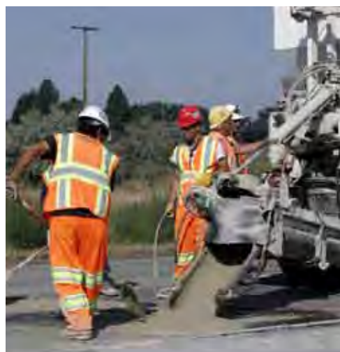
Granite NW Inc. crews place concrete over dowel bar slots on I-82 near Sunnyside in July.
