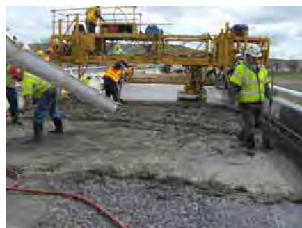
Pouring a 1.5 inch thick concrete overlay.
