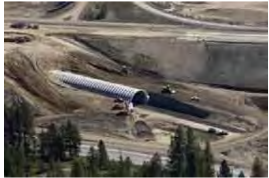
A tunnel will carry trains under the North Spokane Corridor, eliminating conflicts and delays for both freight rail and vehicle traffic.
