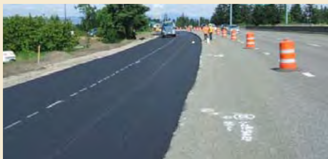
The lengthened SR 500/ I-205 interchange merging lane under construction.
