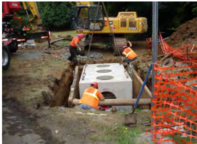
Installation of oil-water separator at the I-5 Gee Creek Rest Area, Clark County.
