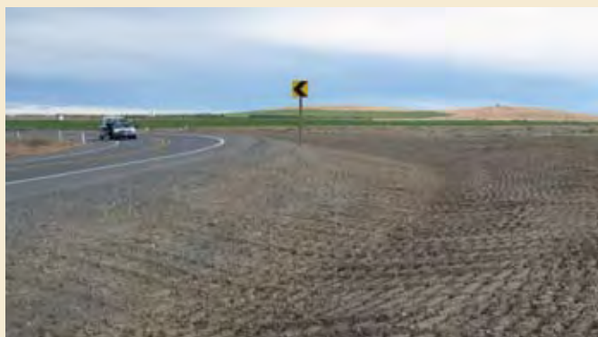
The flattened slope adjacent to this curve is expected to reduce severity of run-off road collisions in the area.
