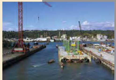
On August 1, the final two pontoons were floated out of the graving dock.
