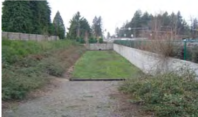
Bioinfiltration swale on SR 500 in Vancouver, Washington.
