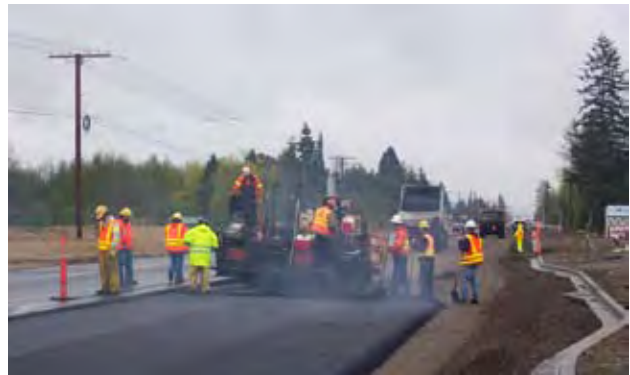
Crews apply HMA as part of the SR 539 - Horton to Ten Mile road project north of Bellingham in early 2008.
