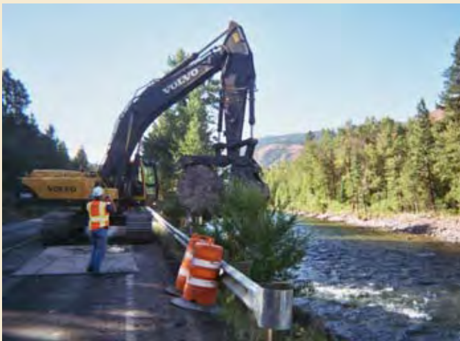
SR 410 along the Naches River. Increased flows from snow melt and winter weather promoted erosion along the river bank, affecting the highway in years past.
