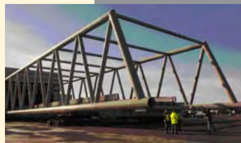
The second of two transition trusses was completed in December.
