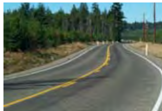
Example of chip seal roadway surface.
