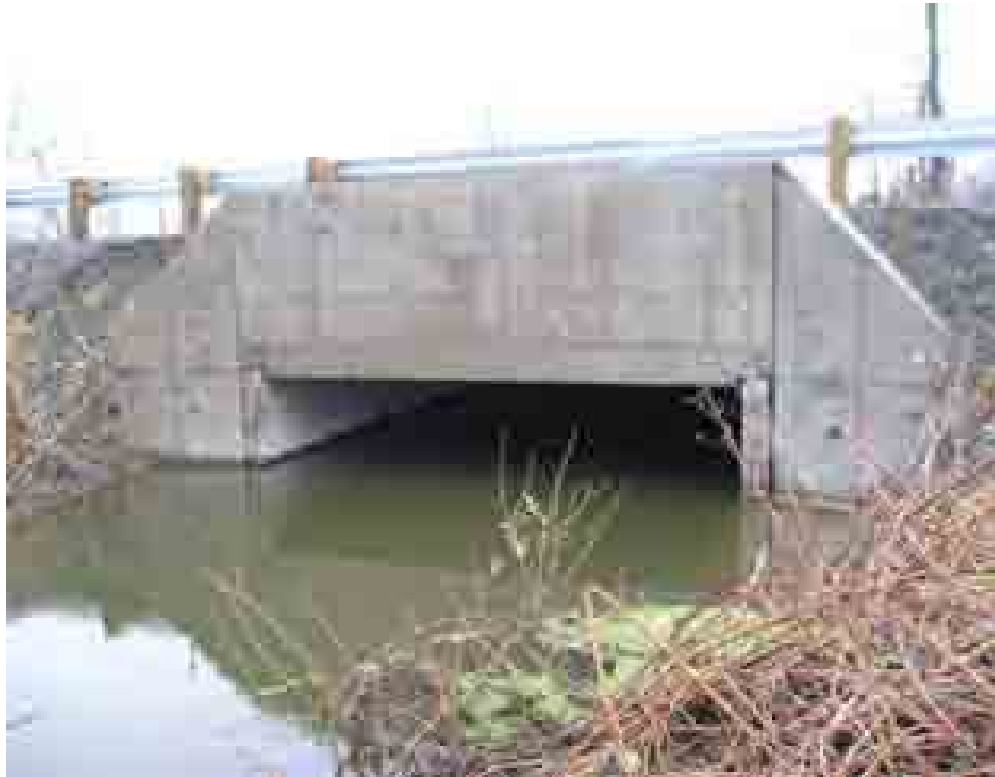
Figure 35. A 4.6 m wide concrete box culvert with a natural streambed material throughout was installed in place of the double pipes during a 2006 SR 9 road realignment project improving fish access to over 3,000 m of up-stream habitat for coho salmon and resident trout.
