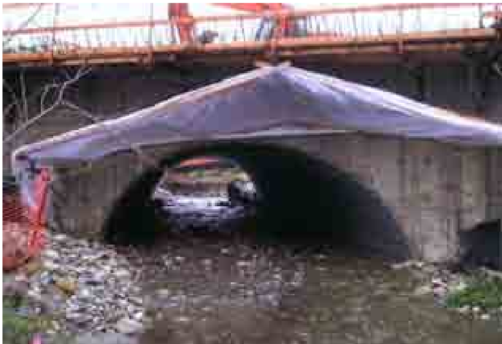
Figure 32. A 4.6 m wide structural plate steel squash culvert with a natural streambed material throughout the culvert was installed in place of the undersized concrete culvert improving fish access to over 1,800 m of habitat for for coho salmon, and steelhead, searun cutthroat, and resident trout.
