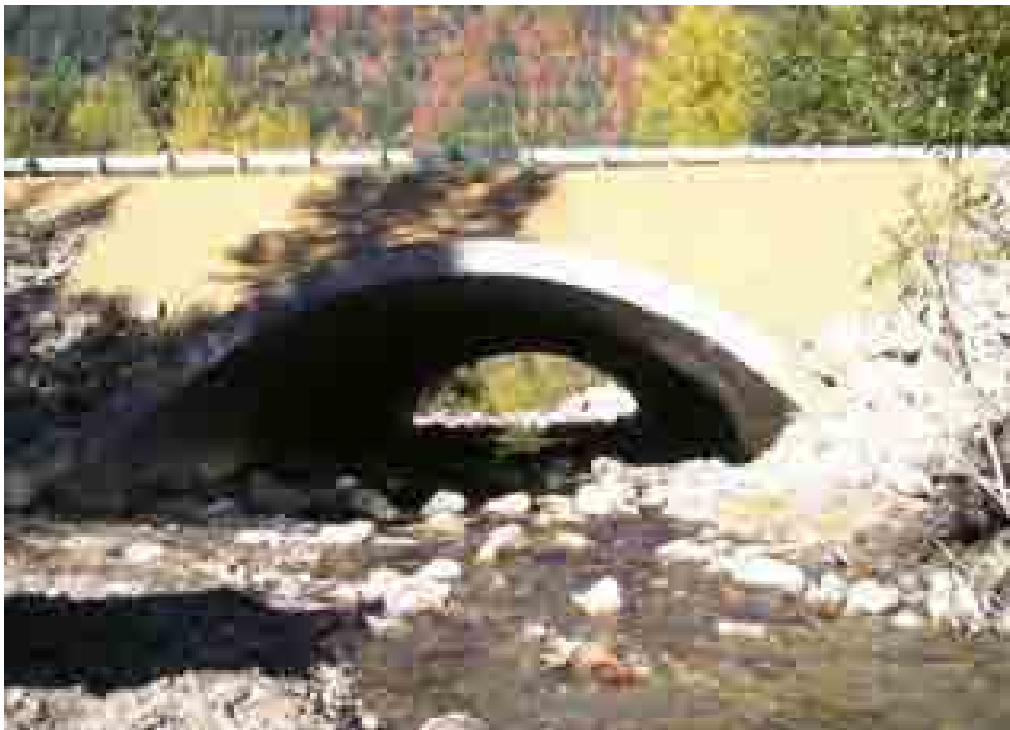
Figure 29. The 2006 project replaced the undersized culvert with a bottomless structural plate arch with natural streambed material placed throughout the culvert. The new crossing restores access to over 11,500 m of habitat to chinook salmon, and steelhead, resident cutthroat, and bull trout.
