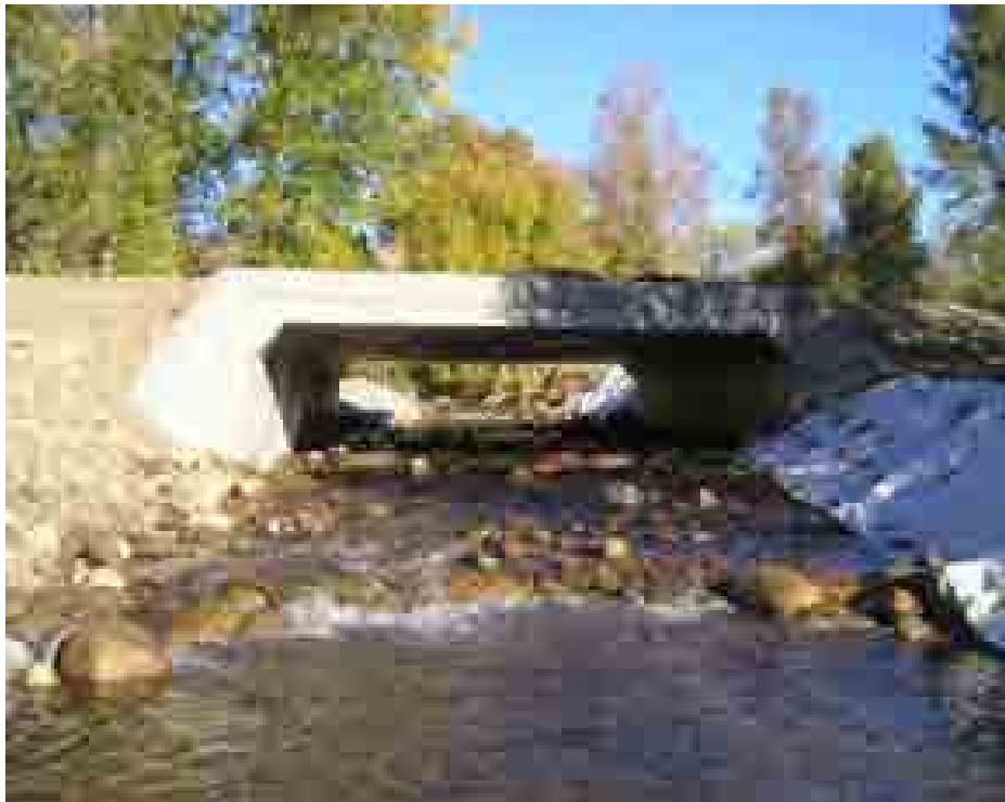
Figure 11. The Beaver Creek culverts were replaced in 2006 with a 7.93 m wide concrete arch culvert through I-4 project. The new culvert provides better access to almost 93 km of habitat to coho and chinook salmon, and steelhead, resident cutthroat, and bull trout.
