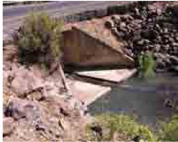
Figure 16. A 3 m wide concrete box culvert was a barrier due to excessive water velocity.
