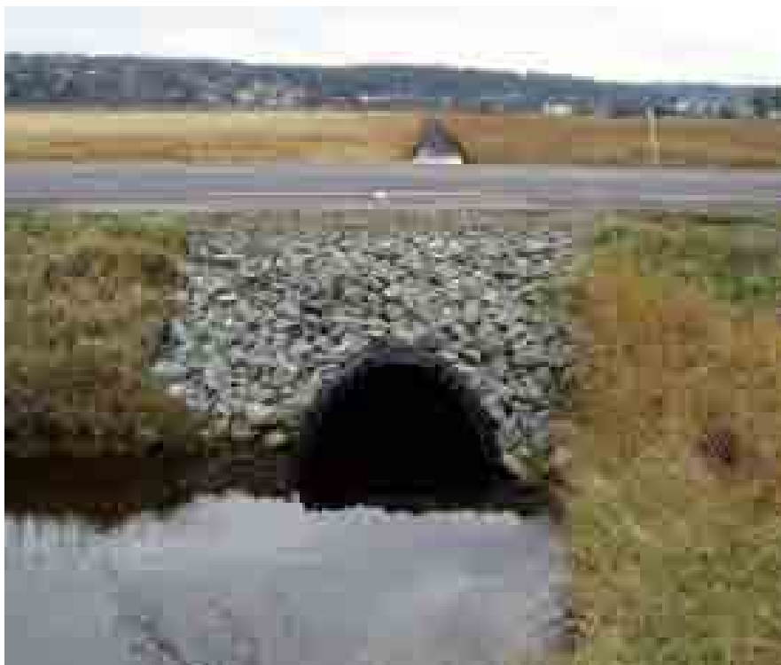
Figure 59. In 2006, WSDOT replaced the culvert with a 1.22 m wide plastic pipe that is passable to fish. Over 500 m of habitat for chum and coho salmon, searun cutthroat and resident cutthroat trout exists upstream of the new culvert.
