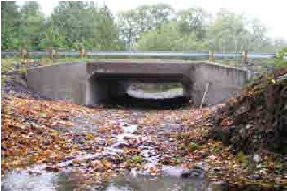
Figure 26. This I-4 funded project replaced the barrier culvert with a bottomless concrete arch with natural streambed material throughout the culvert. The new culvert improves passage to coho salmon, and steelhead, searun cutthroat and resident cutthroat trout to 3,700 m of upstream habitat.
