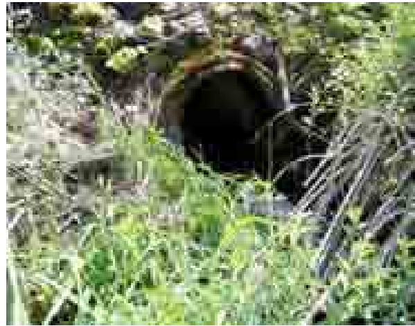
Figure 31. A round, 0.60 m wide concrete culvert was a velocity barrier. The culvert was equipped with 3 downstream controls to temporarily backwater the culvert and provide fish passage.
