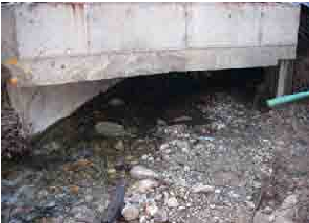
Figure 47. A 3.51 m wide concrete box culvert was installed in 2006 replacing the undersized concrete pipe. The new culvert is set at a 0% slope and has natural streambed material throughout, improving fish passage to over 1,544 m of habitat. Fish species that will benefit from the new culvert include coho salmon, and steelhead, resident cutthroat, and searun cutthroat trout.
