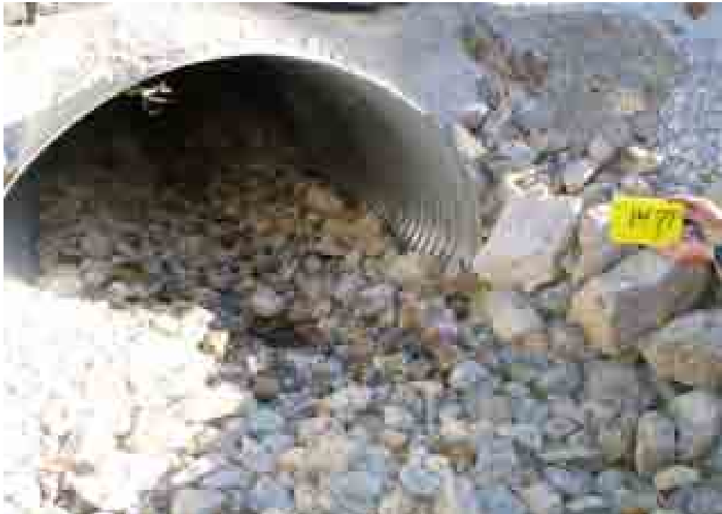
Figure 53. WSDOT replaced the barrier culvert with a 2.4 m wide, corrugated steel culvert, restoring the habitat connection between 8,000 m of potential habitat upstream and the Pend Oreille River downstream for resident cutthroat trout. The new culvert was a part of a 2006 Safety and Mobility project where WSDOT widened the existing two-lane road to a four-lane road.
