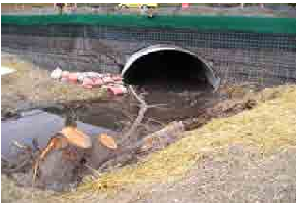
Figure 41. Eight fish passage barriers are slated for replacement during a SR 305 widening project. Four fish passage barriers on South Fork Dogfish Creek have been replaced to date with 100 % passable culverts. Installed in 2006, this new, steel pipe is 2.8 m wide and it has natural streambed material placed throughout. This will provide unimpeded fish passage to over 400 m of potential habitat for coho and chum salmon, and steelhead, searun cutthroat, and resident cutthroat trout.
