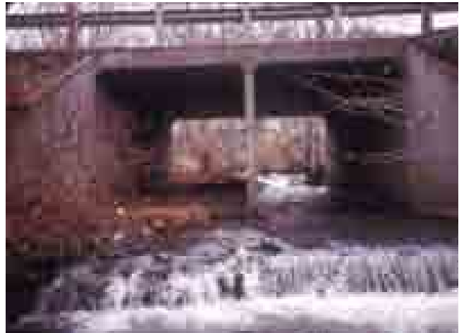
Figure 19. A 3 m wide concrete box culvert was a partial barrier to fish passage due to an 0.51 m water surface drop.
