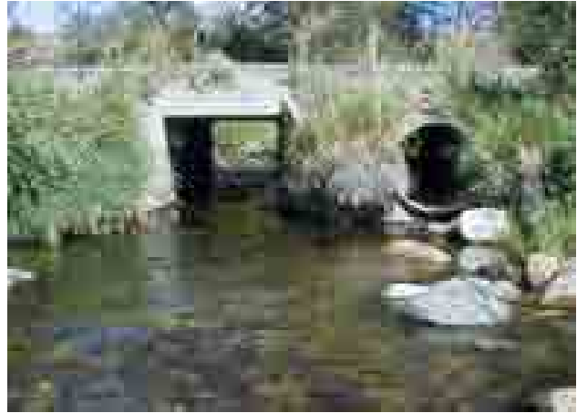
Figure 10. A double culvert crossing consisting of 1.83 m wide, concrete box culvert and a 1.22 m round corrugated aluminum culvert was identified as fish passage barrier due to excessive water velocity.
