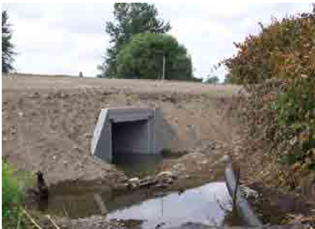
Figure 38. Fish passage at this crossing was addressed in 2006 during the SR 9 realignment project. WSDOT replaced the small steel culvert with a 4.6 m wide concrete box, improving resident cutthroat trout's access to 700 meters of potential habitat upstream while improving drainage.
