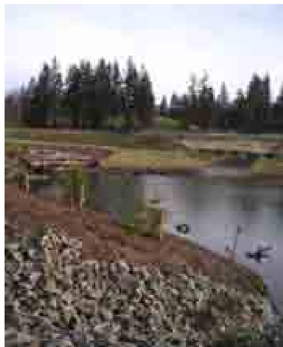
Figure 65. During a 2006 widening project this crossing was eliminated. Fish access to and from Little Bear Creek is available through a 100% passable culvert a little further south on SR 9 - at a milepost 0.88. Along with culvert abandonment, habitat enhancement work was done on this creek, such as addition of woody debris, re-vegetation of stream banks, and realignment of the old streambed to simulate a natural meandering channel.
