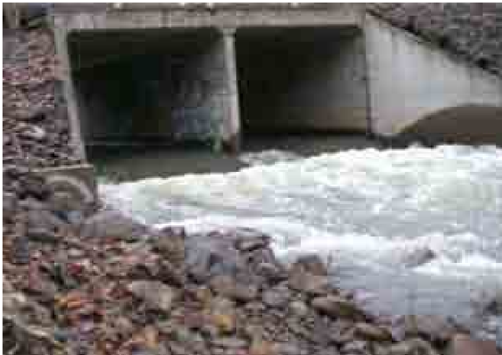
Figure 20. In 2006, WSDOT removed the apron at the mouth of the culvert and re-poured it at a lower elevation. Two weirs were mounted on the new apron to trap bedload, while gravel and rubble was added to floor to add roughness. Wing walls were reworked to provide additional support. The project was funded through the I-4 program. Coho salmon, steelhead trout and resident cutthroat trout will benefit from improved access to over 6,200 m of habitat upstream.
