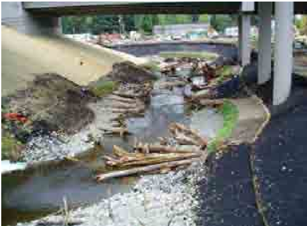
Figure 56. As part of the SR 18 widening project, WSDOT replaced a baffled culvert with a bridge. The old culvert was blocked off and the flow rerouted to a new channel equipped with log controls and large woody debris. The bridge improves access to over 3,300 m of potential habitat for sockeye and coho salmon and resident cutthroat trout.
