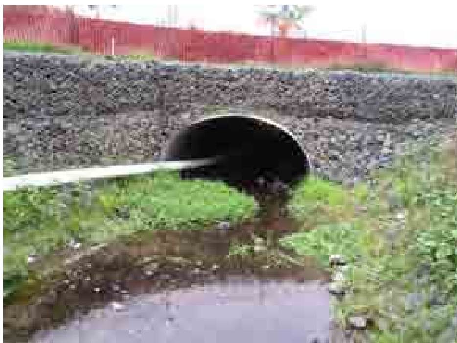
Figure 50. The new, 2.6 m wide corrugated steel culvert was installed in place of the old concrete pipe in 2006 during a road-widening project. Coho and chum salmon, and steelhead and resident cutthroat trout will benefit from almost 600 m of potential habitat upstream of this crossing.
