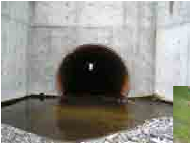
Figure 62. In 2006, WSDOT replaced the old pipe with a 1.7 m wide concrete pipe. Over 1,200 m of habitat for coho salmon, and searun cutthroat and resident cutthroat trout exists upstream of the new culvert. The new culvert was installed at a slope of less than 1% and in such a way as to gain an additional 250 feet of stream habitat downstream of the culvert. The photo on the bottom right shows a newly created channel equipped with concrete controls and large woody debris.
