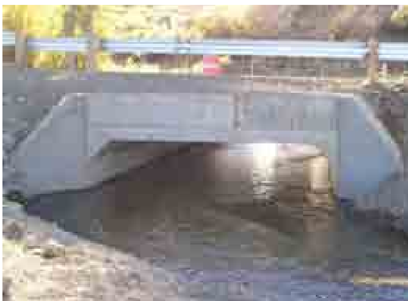
Figure 14. In 2006, the two steel culverts were replaced with a 4.57 m wide concrete arch stream simulation culvert. The I-4 project included another barrier culvert replacement at Beaver Creek (see Figures 9-11). This project improved fish access to 12,290 meters of habitat upstream for chinook and coho salmon, and steelhead, bull, and resident cutthroat trout.
