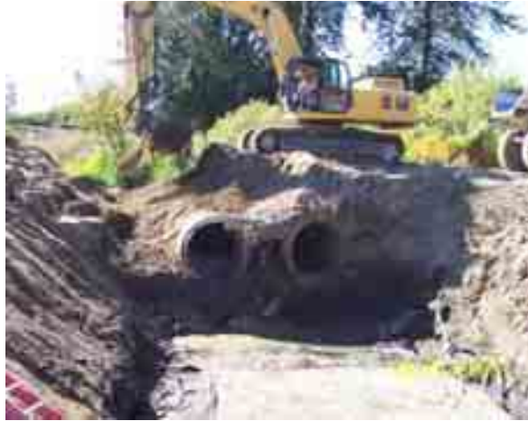
Figure 34. Two round, 1.22 m concrete culverts were undersized creating a velocity barrier.
