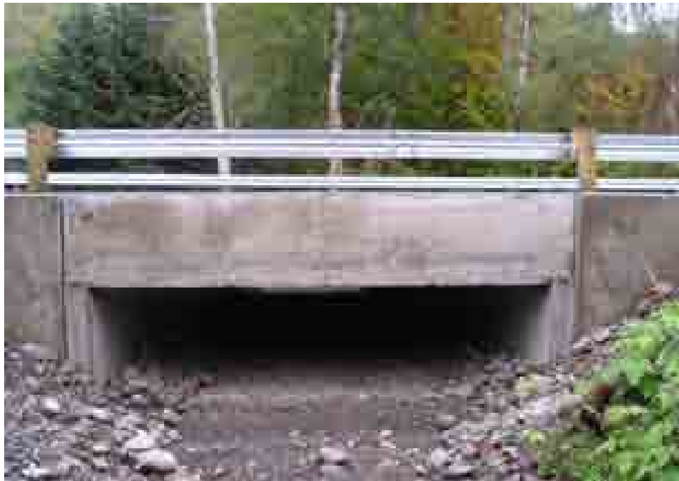
Figure 23. A 4.6 m wide concrete box culvert with natural streambed material throughout the culvert was installed in place of the double pipes improv- ing fish access to over 3,000 m of habitat for coho salmon and resident cutthroat trout.
