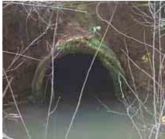
Figure 64. A 0.76 m wide corrugated steel round culvert was too small for the stream.
