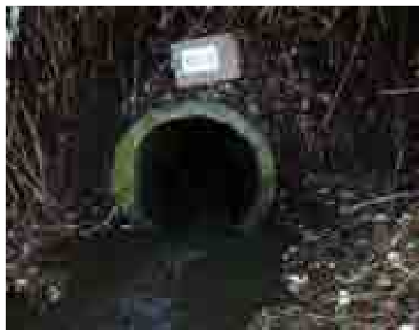
Figure 46. A 0.61 m wide, round concrete culvert was evaluated as a barrier due to a 3.8% slope.
