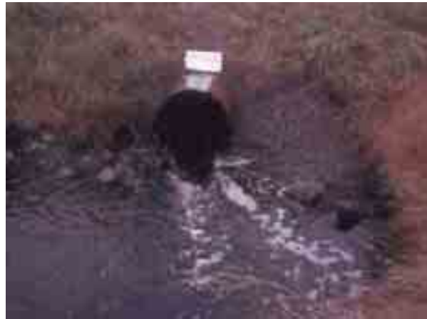
Figure 58. A 0.76 m wide corrugated steel round culvert was undersized.
