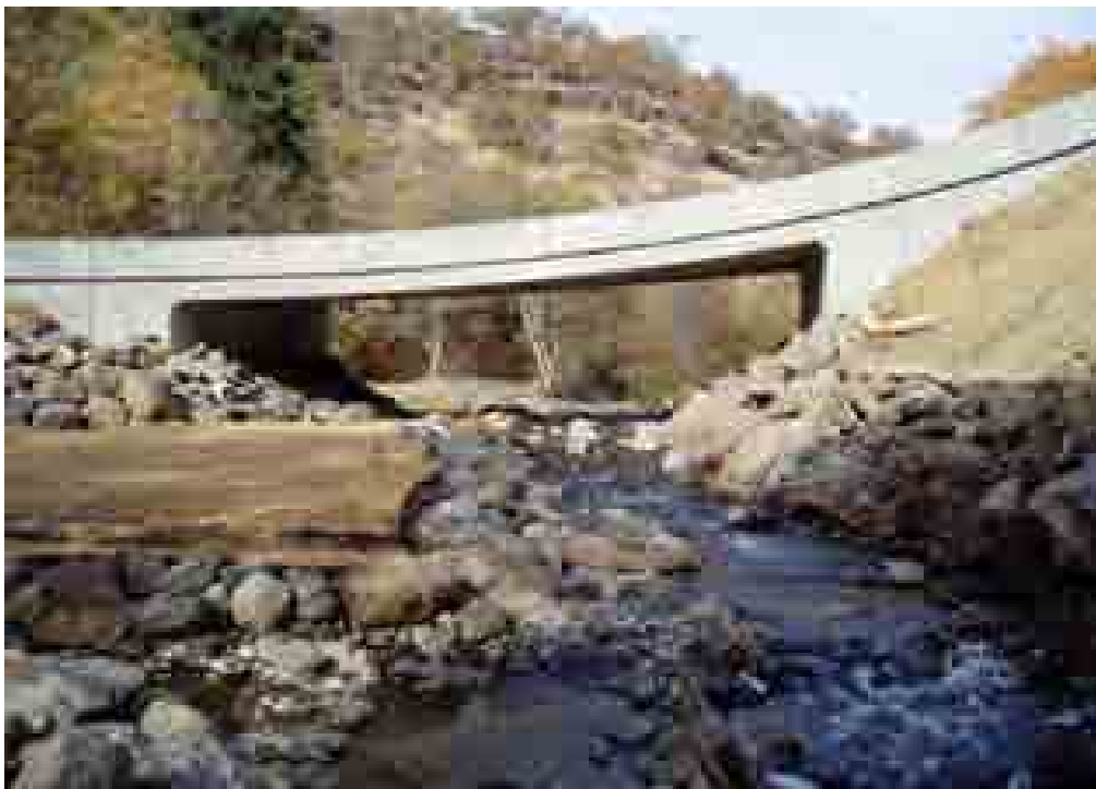
Figure 17. In 2006, the box culvert was replaced with a full-span, 18 m wide bridge, providing 36,671 m of upstream habitat available for coho salmon, and steelhead, bull, and resident cutthroat trout.
