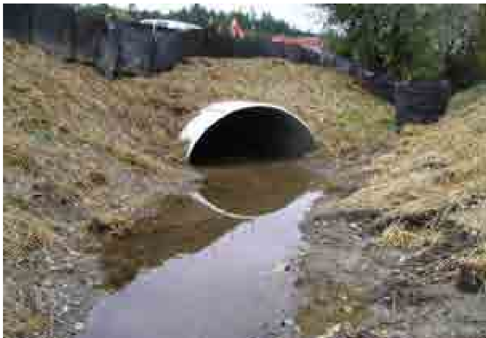
Figure 44. A 2.85 m wide structural plate steel culvert was installed in 2006 replacing the under-sized concrete culvert. The new culvert is set at a slope of less than 1% and has natural streambed material throughout, providing unobstructed fish passage to over 1,000 m of habitat for coho and chum salmon, and steelhead, resident cutthroat, and searun cutthroat trout.
