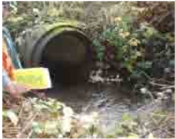
Figure 43. A 0.91 m wide, round concrete culvert was a velocity barrier.
