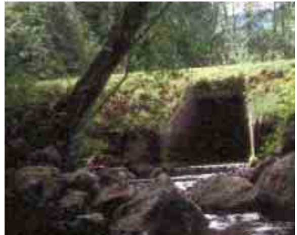
Figure 25. A concrete box culvert, 1.83 m wide was a velocity barrier to fish passage.
