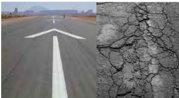
Left: Airport pavement in "Good" condition. Right: Airport pavement in "Poor" condition.
