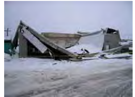
WSDOT's Wandermere maintenance facility collapsed under a heavy snow pack in Spokane.
