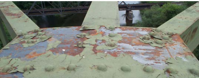
Crews will repaint all of the steel on the truss of the SR 18 Green River (Neeley) Bridge near Auburn in summer 2015. This will protect the steel for another 20 years and help preserve the bridge’s structural integrity.
