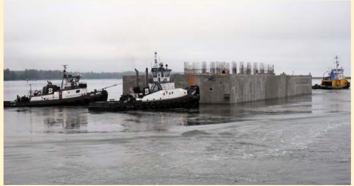
Tugboats tow one of the pontoons for the SR 520 floating bridge replacement from the casting basin in Aberdeen to Lake Washington.
