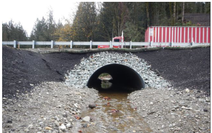
WSDOT repaired this culvert along with five others along State Route (SR) 530 after a landslide in March of 2014. These repairs, part of WSDOT's overall effort to repair SR 530 after the landslide, corrected three documented fish passage barriers.
