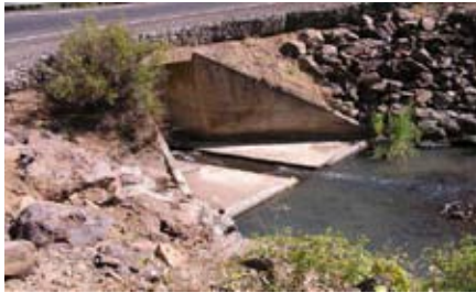
BEFORE: SR 142 near Goldendale and Bowman Creek. A 9 foot box culvert was a velocity barrier during high flows and prevented fish passage.
