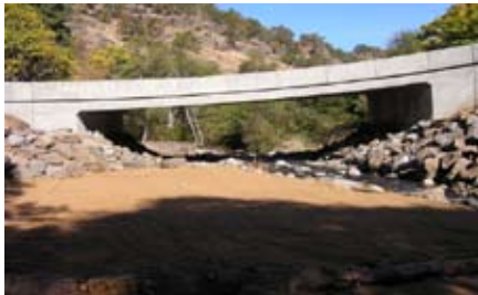
AFTER: A new 60 foot bridge restored fish passage for coho salmon, steelhead, bull and resident cutthroat trout.
