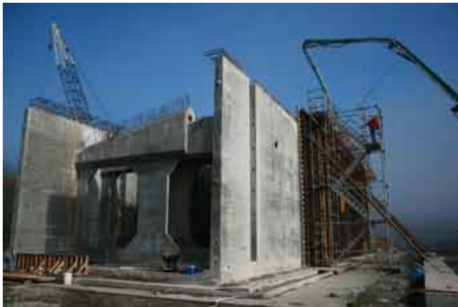
One of the test pontoons constructed in preparation for the SR 520 floating bridge replacement project.
