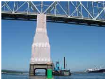
SR 433 Lewis and Clark – The containment area during Phase 2 of construction to clean and paint the piers in the Columbia River and bridge towers on the Washington side.
