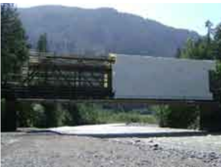
SR 542 Nooksack River – Crews have more than half of the containment system required to complete the bridge painting in place.
