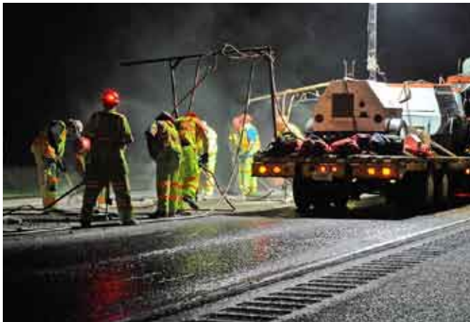
Crews chipping out slots for replacement dowel bars on I-5 near Martin Way in Lacey
