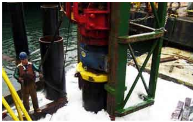
Impact-pile installation at WSDOT's Eagle Harbor facility on Bainbridge Island. A 'bubble wall' is being used to help absorb underwater noise.
