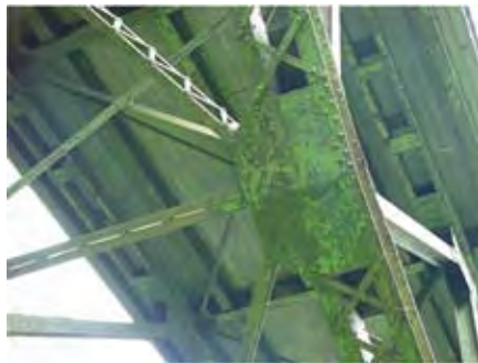
Condition State 2: Paint is failing but no steel exposure.
