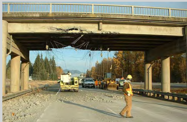
On 10/31/2007 a truck pulling an oversized load on I-90 struck an overpass near Easton. The overpass was damaged beyond repair and was removed on 11/1/2007. A new bridge was completed on 12/15/2007.
