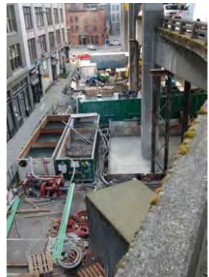
View of the new concrete surrounding the bridge footing on the Alaskan Way Viaduct.
