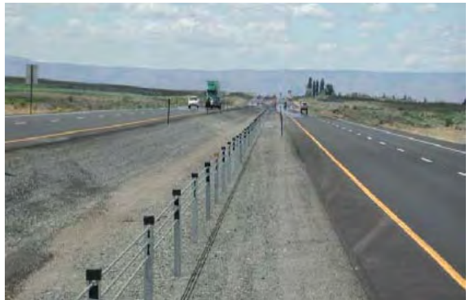
WSDOT installed 43 miles of cable median barrier in 2007, bringing the statewide total to 177 miles.
