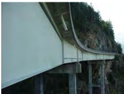
Condition State 1: Paint is in good condition.
