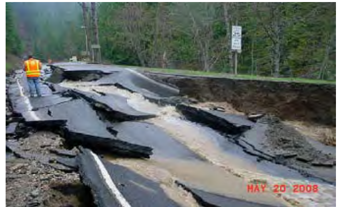
A WSDOT employee looks at the damage done to SR 206 on Mount Spokane just days after the road was washed out.
