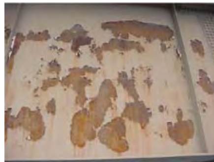
Condition State 3: Paint has failed with steel exposure.
