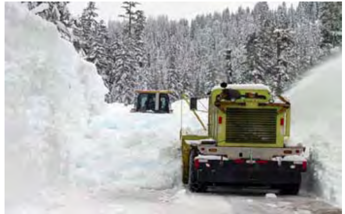
On March 26, 2008, a dozer and snowblower work as a team to clear a path through 18 to 19 feet of snow at milepost 65.4 of Ghost Lake on Cayuse Pass.
