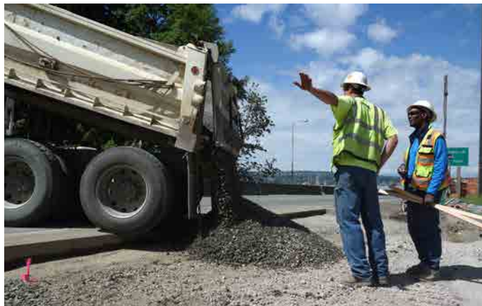
Crushed rock is placed prior to paving a new section of State Route 520.
