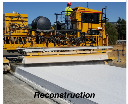
A concrete roadway on I-90 east of Cle Elum undergoes reconstruction in 2015. Concrete reconstruction is the most expensive method for managing pavement, costing $2.5 million per lane mile, but adds 50 years of life to the roadway.
