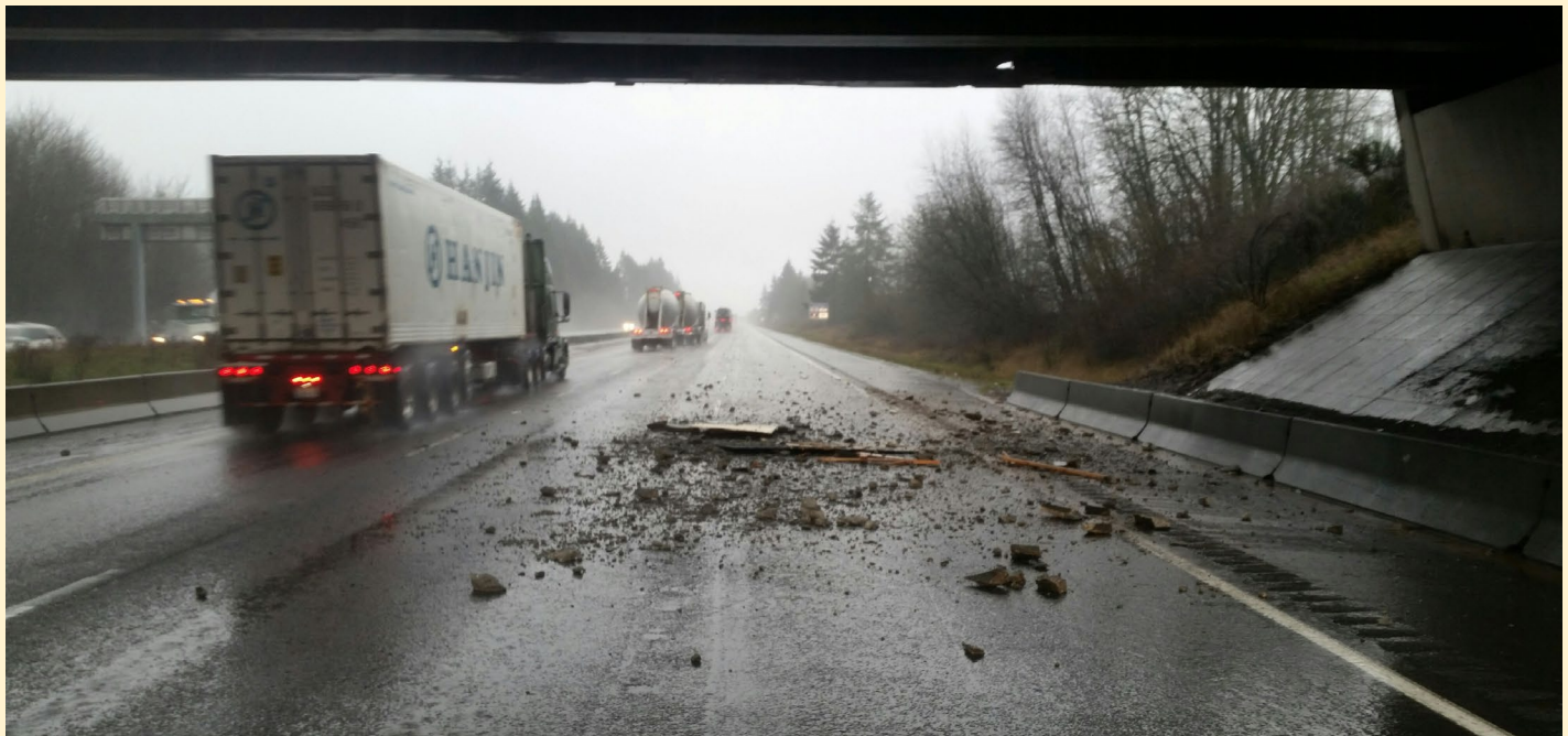
The I-5/Koontz Road overpass was hit by an oversize load in December 2015. WSDOT used emergency procedures to move forward with the repair of two of the four girders that support the bridge.
