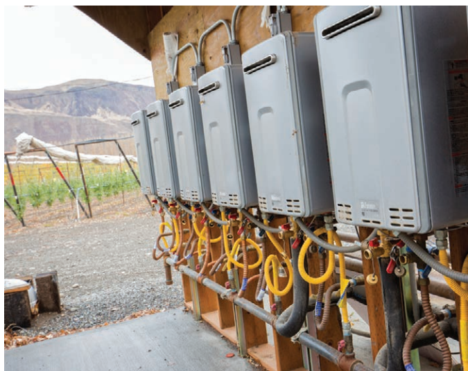
Feigal is experimenting with on-demand propane water heaters to warm a 6-acre block of trees in late winter at Auvil Fruit Company near Vantage. The heaters supply hot water to underground pipes beneath the apple trees in the distance.
