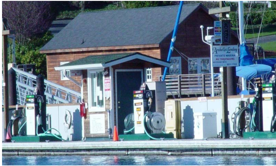
Figure 3.30. Fuel dock in Gig Harbor. Photo: Washington DNR
