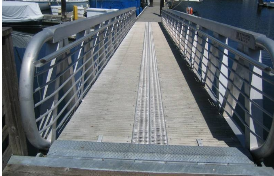
Figure 3.26. Partially grated walkway on Gig Harbor. Photo: Washington DNR
