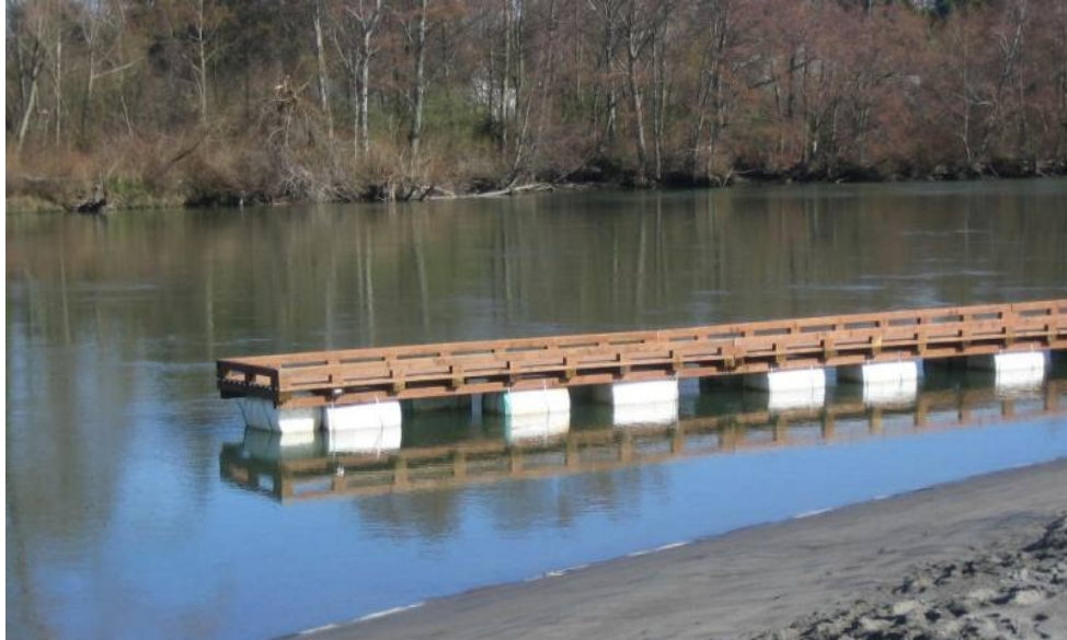
Figure 3.27. Flotation made of foam-filled white plastic tubs on the Skagit River. Photo: Washington DNR
