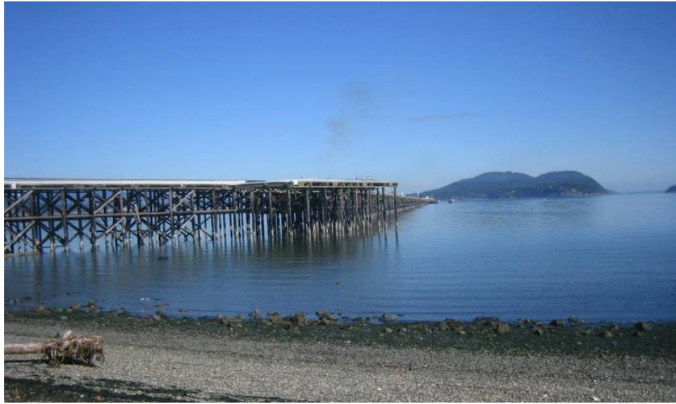
Figure 3.24. Terminal on Fidalgo Bay. Photo: Washington DNR
