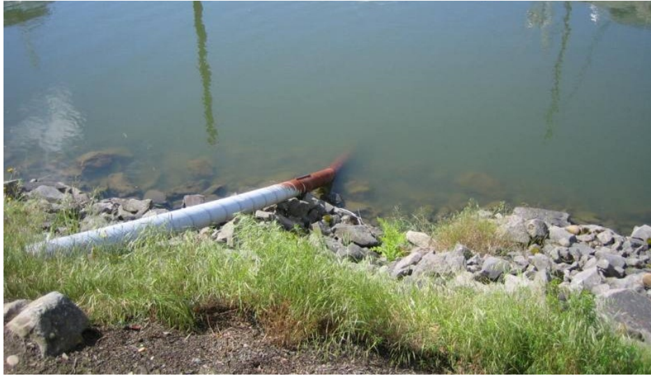
Figure 3.32. Outfall on the Columbia River. Photo: Washington DNR
