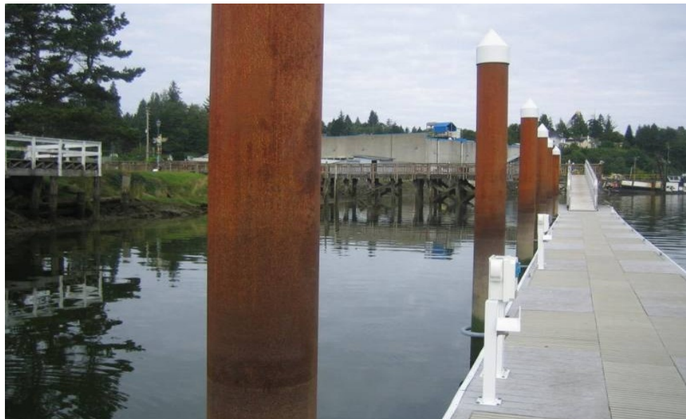
Figure 3.28. Steel pilings on the Willapa River. Photo: Washington DNR
